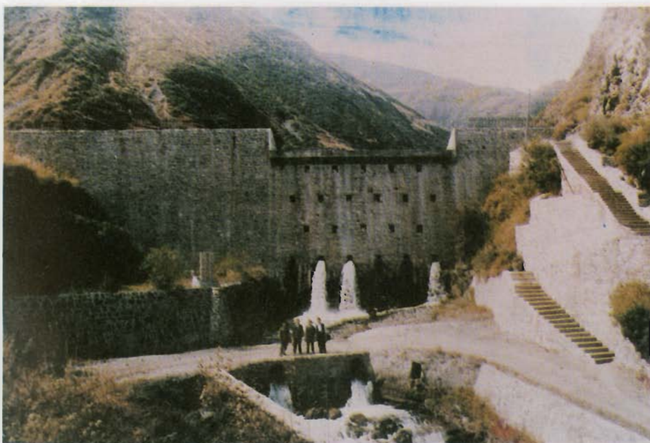
Plate 6: An Arched - Foundation - Masonry - Sifter Type Checkdam, 23m high, in Babuli Ravine, Jinchuan County, Sichuan - Li Deji
