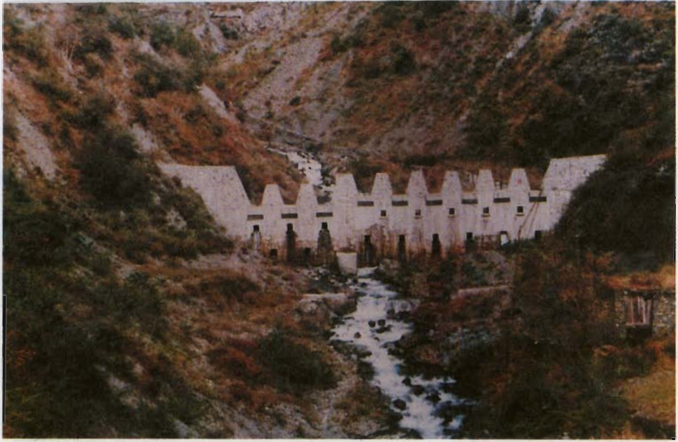
Plate 7: A Sawtooth-Type Checkdam, 10m High in the Babuli Ravine, Jichuan County, Sichuan - Li Deji
