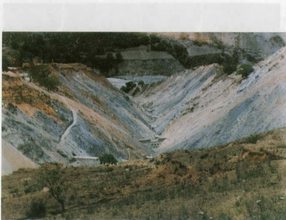
Plate 4: Stepped Checkdams to Control Landslides and Debris Flow in the Daqing Ravine of Daxueshan, Yongbi County, Yunnan - Li Deji
