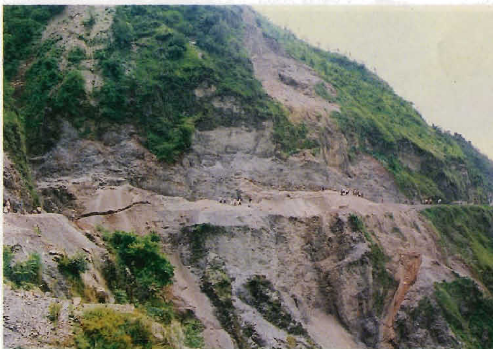
Plate 2: Rockslide in the highly crushed zone near Jhakri Danda, Kanti Rajpath, Central Nepal.
