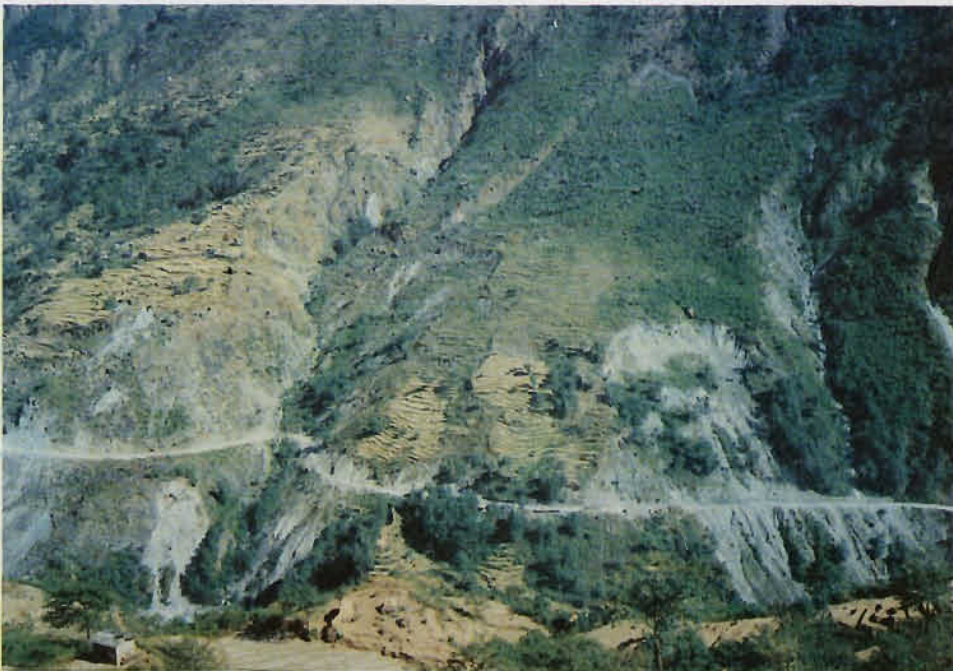
Plate 8: Soil slides at Daklang (about 2km north of Chaku Khola) along the Arniko Highway).
