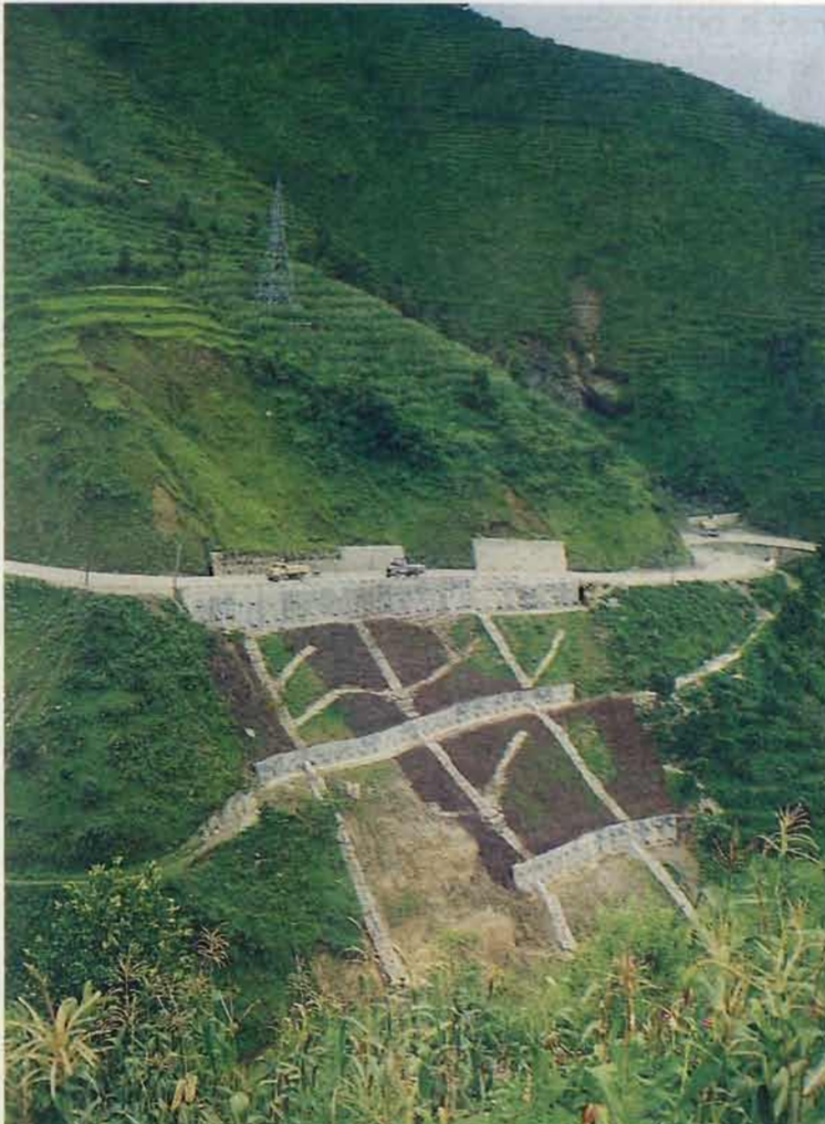
Plate 9: Gully erosion protection work in the Charnawati Valley using concrete lining on the stream floor, to make cascades, concrete retaining structures along the banks, and large tetrapods along the streambed and the banks
