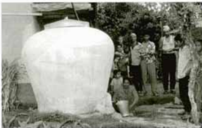
Figure 13: Rooftop rain water harvesting jar in Hokse, Jhikhu Khola watershed
