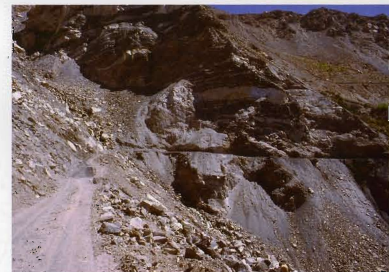
Himalayan roads constantly face the danger of landslides. Here, a 100-meter section of road in Lahaul district slipped away, causing vehicular traffic to detour over 500 kilometers.
