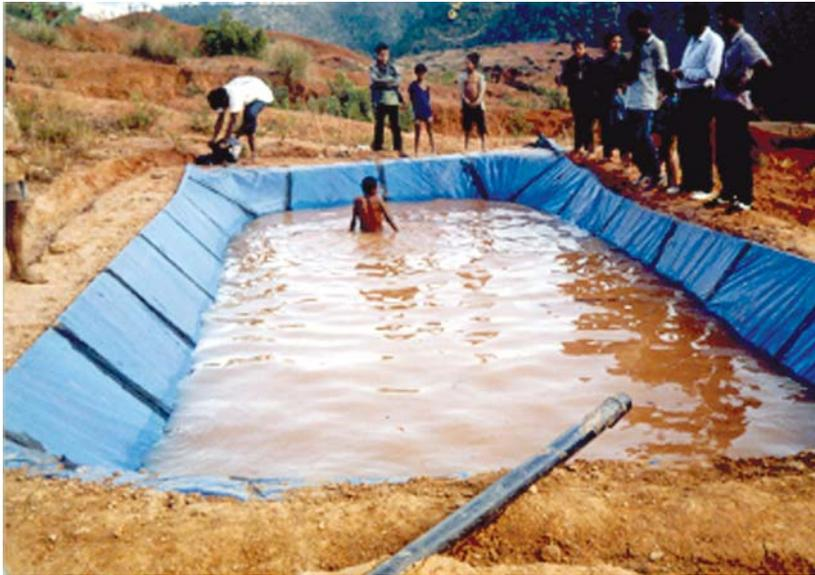
Figure 3.11: A plastic-lined water harvesting pond
