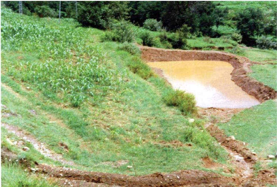
Figure 13.4b: **A pond built to collect water diverted from a rehabilitation site, Pakistan (PFI 1994)**
