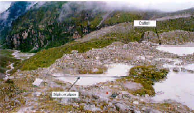
Figure 12.2: Closer view of Tsho Rolpa Glacial Lake mitigation construction site (photograph source DHM 2000)
