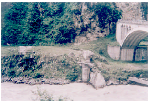
Figure 9.12: Remnant pier of the old bridge damaged by the 1981 GLOF and the new bridge at Phulping along the Nepal–China Highway
