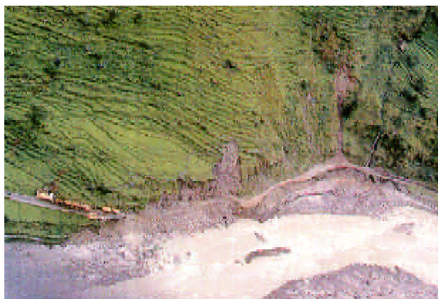
Figure 9.13: The washed out portion of the Kodari Highway (Nepal–China Highway) by the 1981 GLOF
