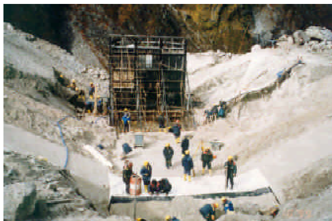
Figure 12.3: Gate structure with partially erected gates. In the foreground geomembrane and geotextile are being laid (photo credit: Shrestha 2000)
