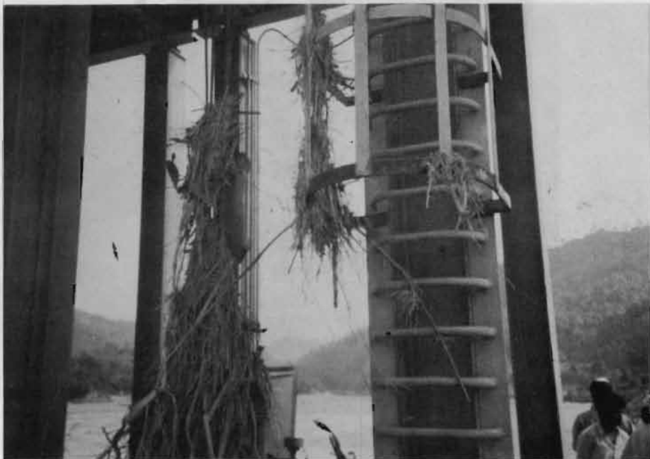
Debris entangled above the gates
