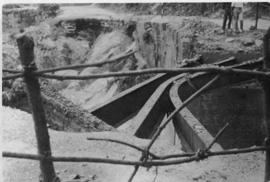
Plate 20: The washed-out bridge at Trikhendi. The steel beams are bent by the debris and boulders passing underneath the bridge. View towards the north-west
