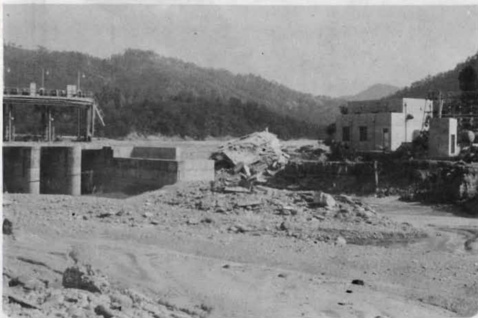
Plate 59: The washed-out control tower on the left bank of the barrage. Notice also that the sediment undersluices and the eastern canal are filled up with gravel. View towards the north
