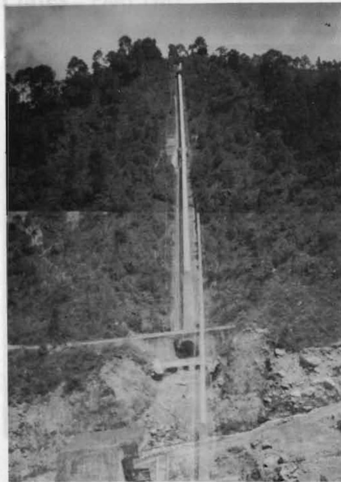
The smashed penstock by the debris flow at Jurikot
