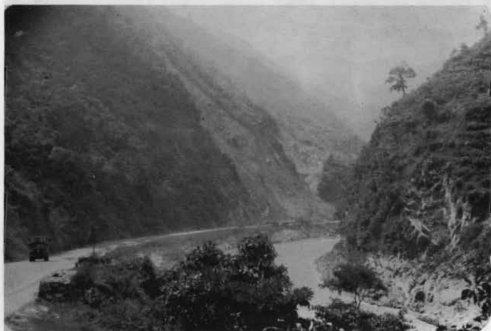
Plate 35: The Jogimara rockslide in slates and limestone. A stone quarry is also seen on the right bank. View towards the south-west
