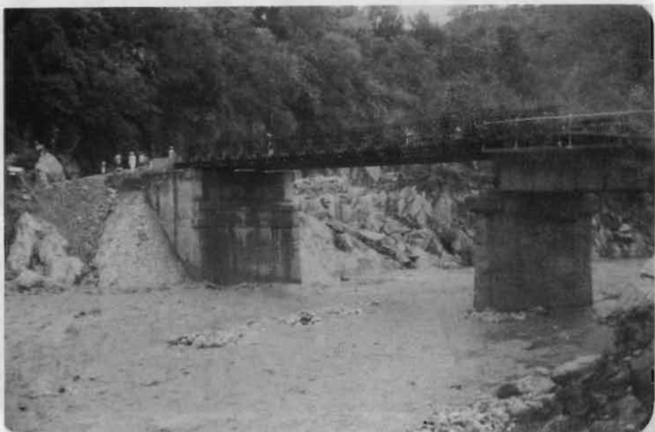
Plate 29: The partially damaged bridge over the Malekhu Khola replaced by a Bailey bridge. View towards the east
