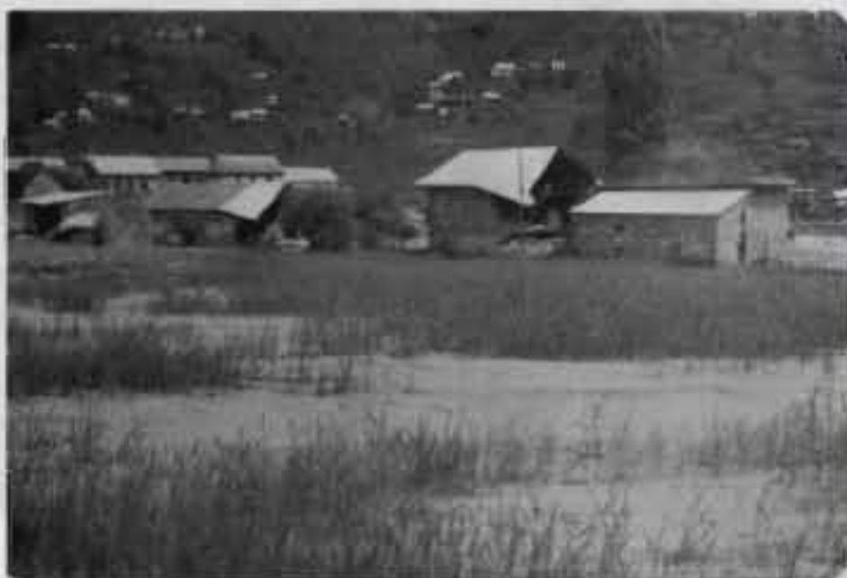
Plate 42: The paddy field in Palung filled up with 0.5 m thick sand. Notice also the damaged houses. View towards the north.
