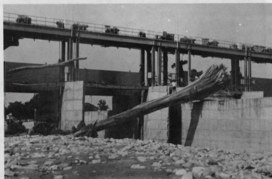
Plate 56: A large tree trunk resting over the dividing wall of the western canal. Notice also another log entrapped in the raised gates. View towards the south
