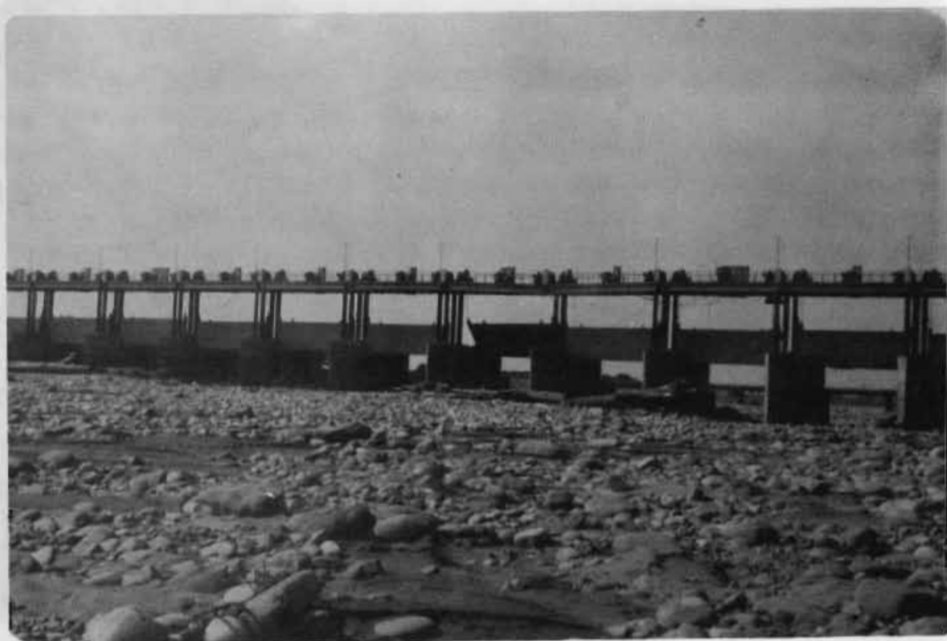
Plate 55: Downstream view of the Bagmati Barrage and the mid-channel bar. Notice a damaged gate (in the centre) and a 33 m long tree trunk. The Bagmati Bridge is seen in the background. View towards the south
