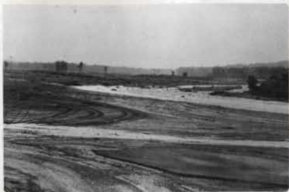
Plate 65: The breached dykes on the right bank of the Manohari Khola. The river shifted to the west and destroyed the cultivated land of the Chitwan Valley
