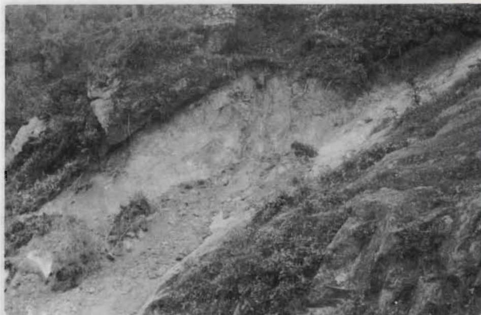
Plate 22: The wedge rockslide on the moderately to highly weathered granite, the Tribhuvan Highway north of Sikharkot. View towards the south
