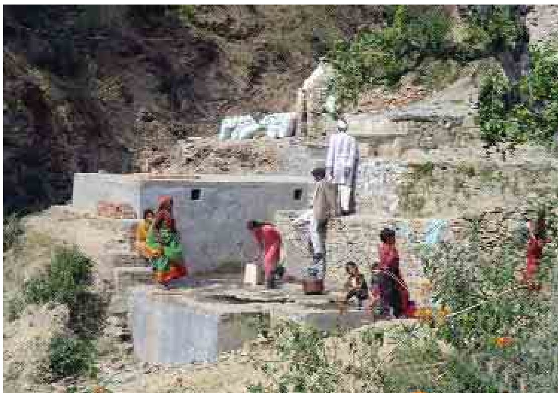
Figure 4.10: Tank and water outlet of the recharged traditional spring in Bajeena, Uttarakhand
