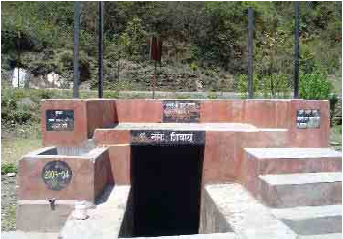
Figure 4.13: Newly-constructed retention tank for traditional pond at Ghagar-Sayawan in HP, India
