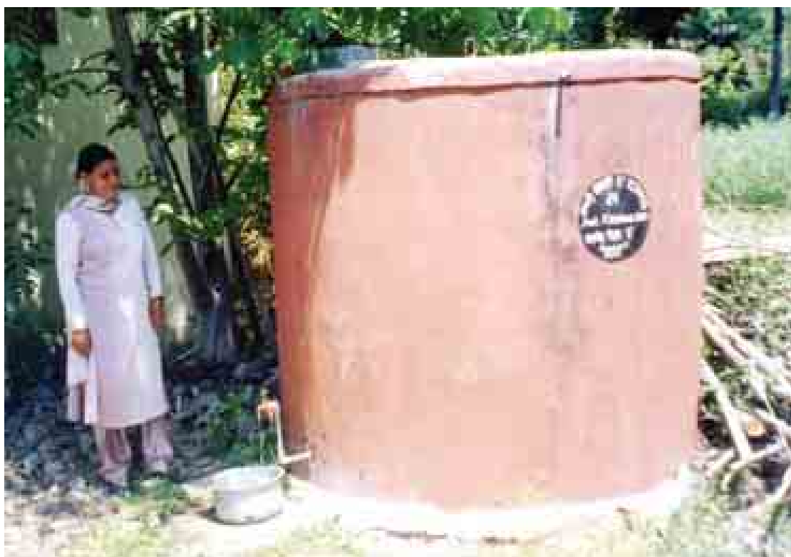
Figure 4.12: Harvesting tank for rooftop rainwater in India
