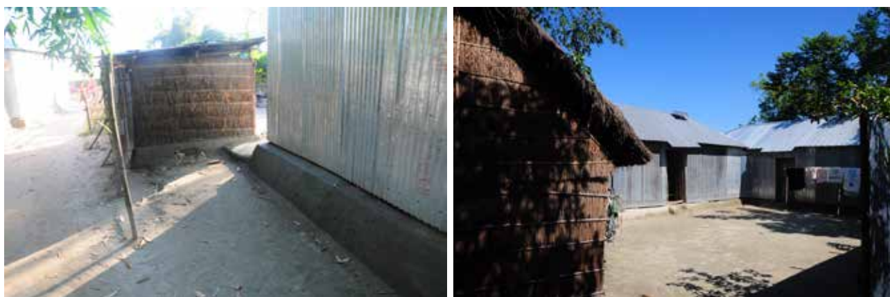
Figure 6: Commonly-built houses with raised plinths in the Teesta basin floodplain and chars
