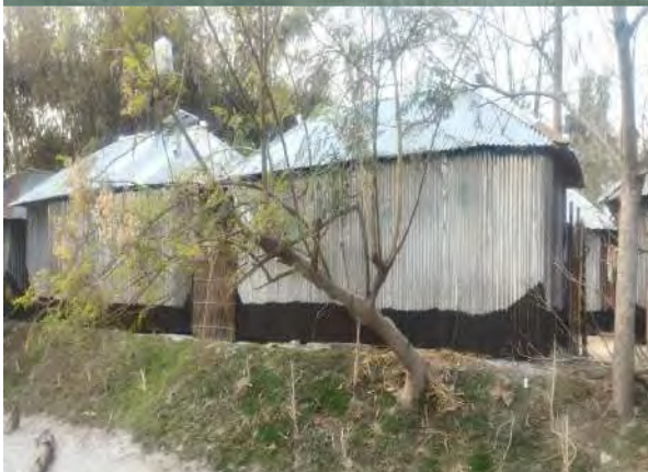
Figure 2: Reconstructed CFR House on a raised plinth with side protection layer of grass and saplings
