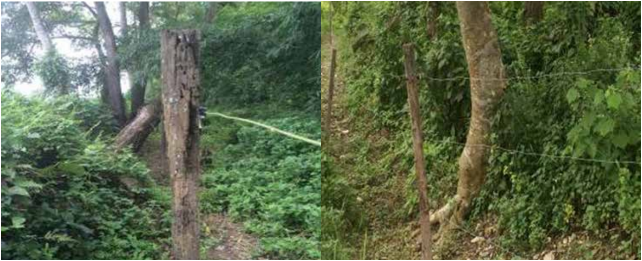
Low quality/rotten wooden poles used as structures for electric fences
