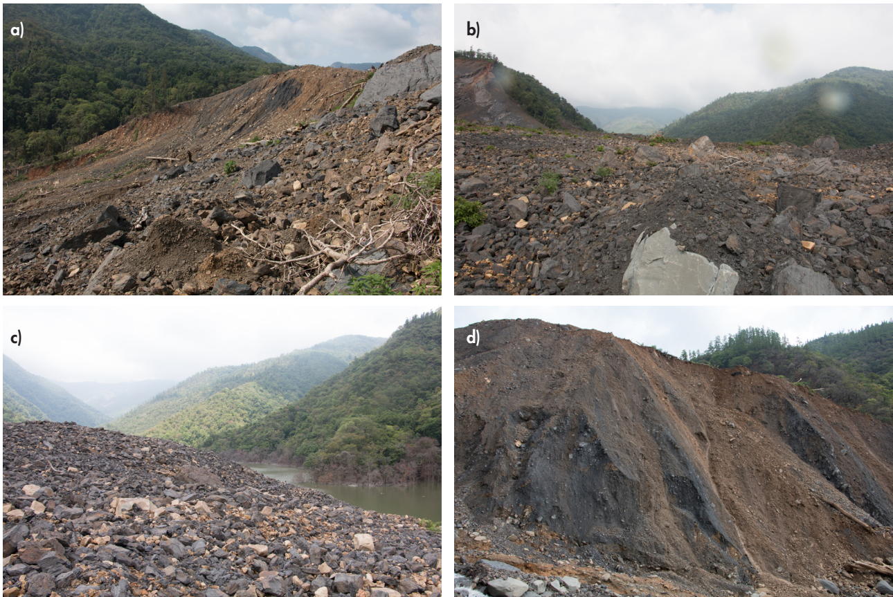
Figure 6: Dam material analysis; a) view from lake to highest crest; b) view from lowest crest toward lake; c) on lower crest at right side of the dam; and d) toe of dam.
