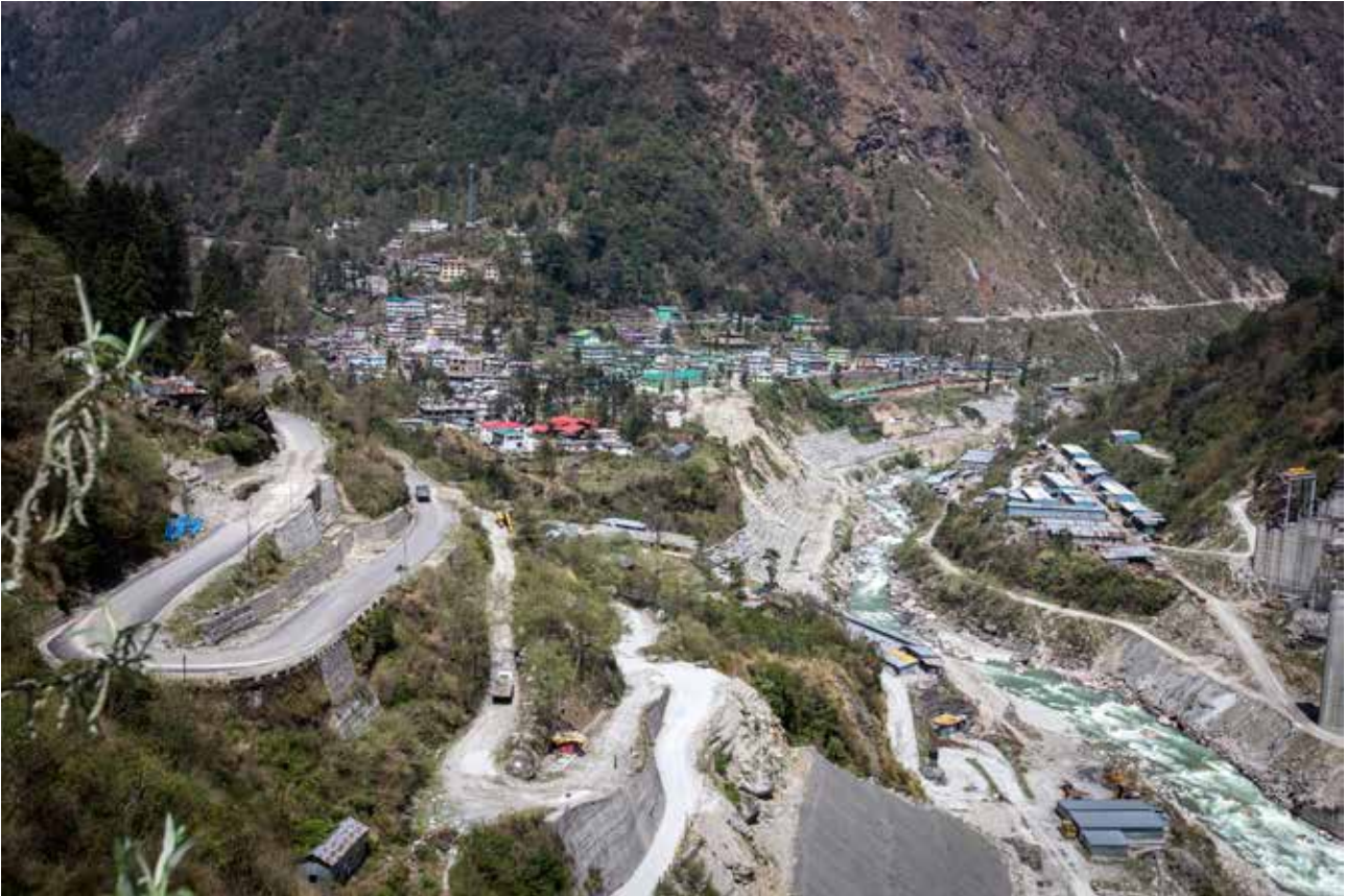
Teesta III dam wall construction at Chunthang, Sikkim (India)
