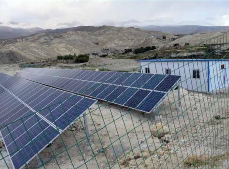
Lomanthang, a trekking destination in Upper Mustang, has a solar microhydro mini-grid system. A 29 kW microhydro plant supplies electricity to 190 households in Lomanthang VDC. In 2015, a 70 kW solar power station with 300 solar panels was installed to fulfil electricity requirements in the winter. The community now has round-the-clock electricity. Locals use less than 30 % of the grid system's full capacity to fulfil their lighting, cooking, and entertainment needs.
