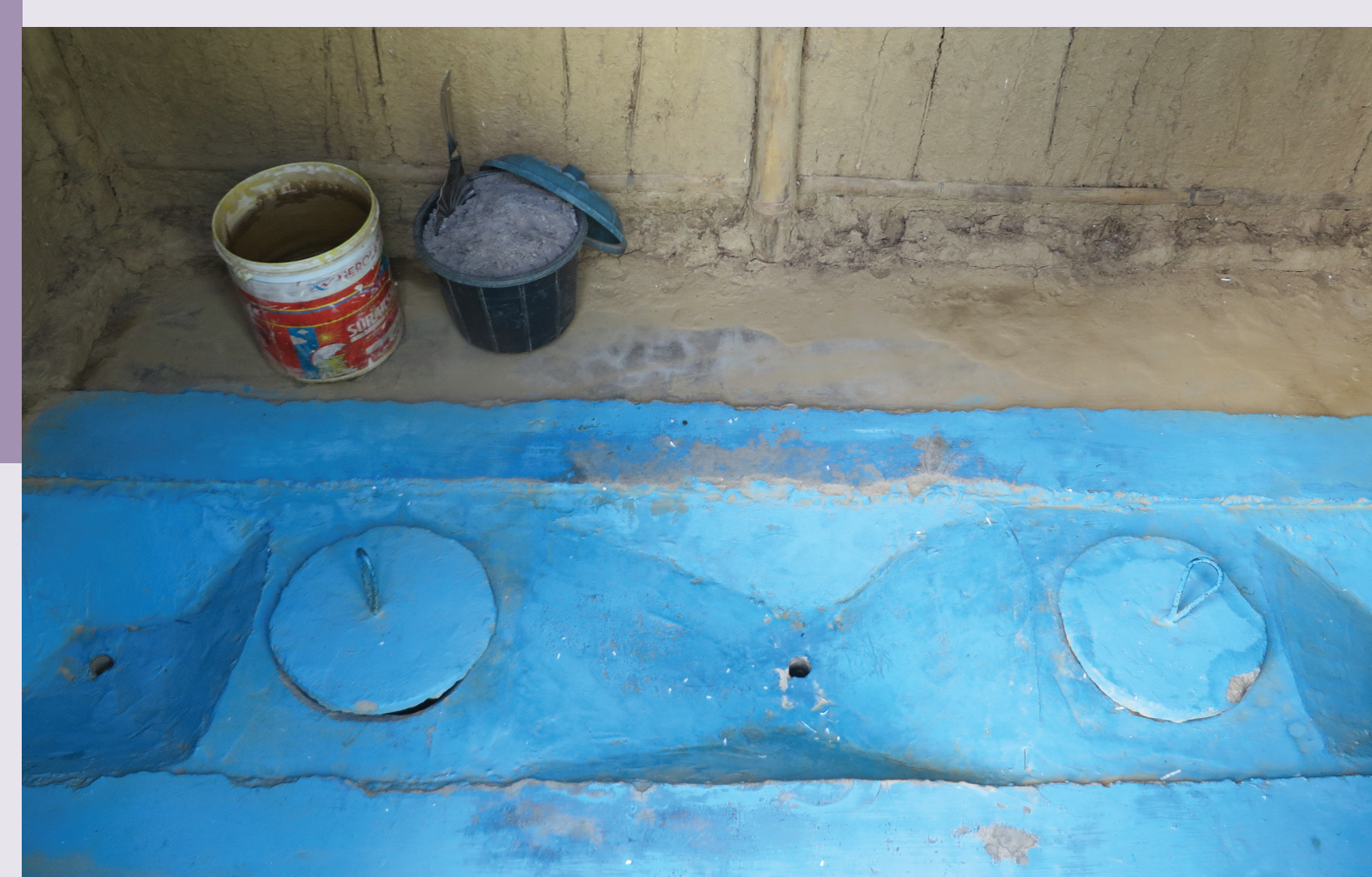
Figure 1: Illustration of urine and faeces outlet of the Eco-san
