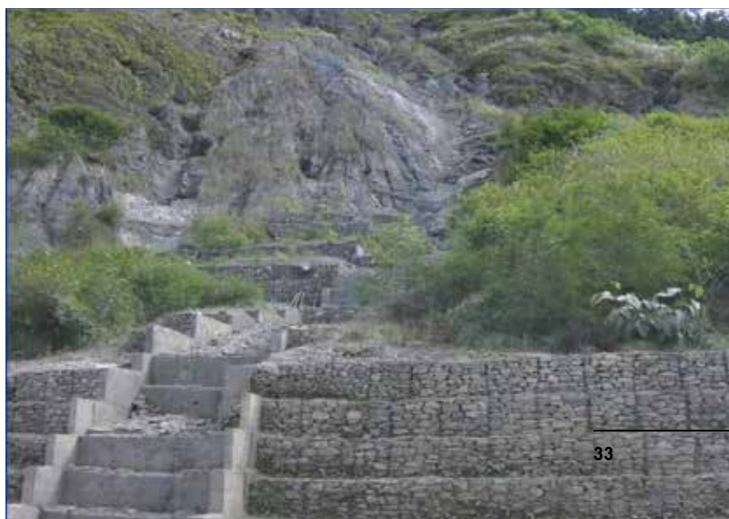
Figure 18: Civil engineering and bioengineering were used together to stabilize the famous Krishnavir landslide west of Kathmandu
