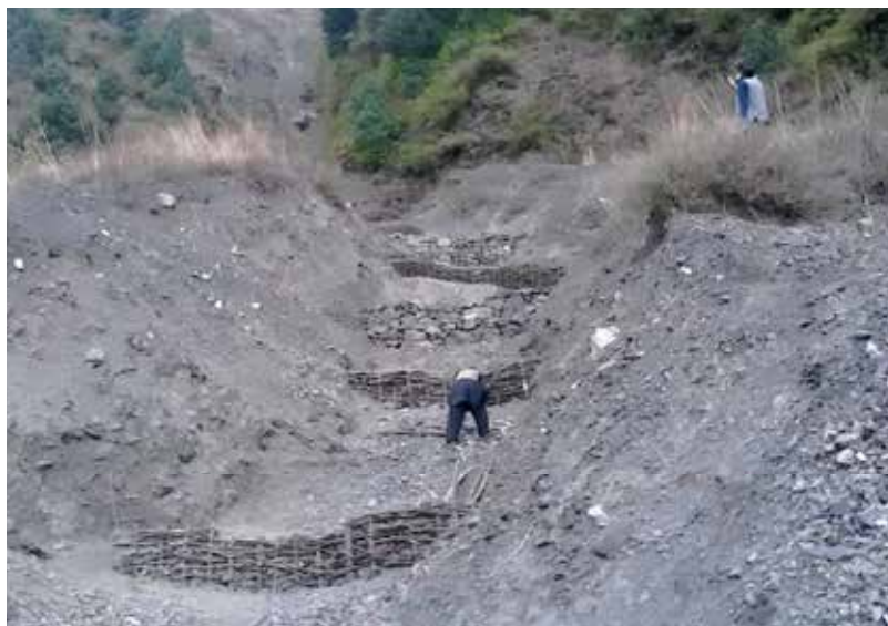
Figure 21: Rehabilitation of landslide sites in Bagnota using local materials
