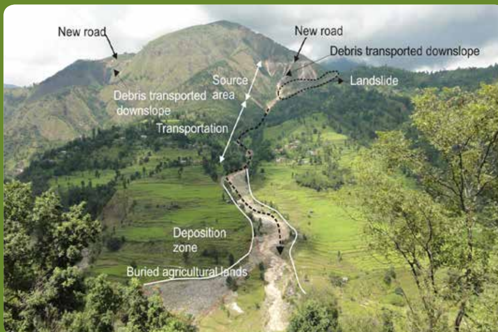
Figure 22: Road construction in Arukharka VDC, Syangja District, in western Nepal is seen destabilizing hill slope and resulting in ensuing hazard
