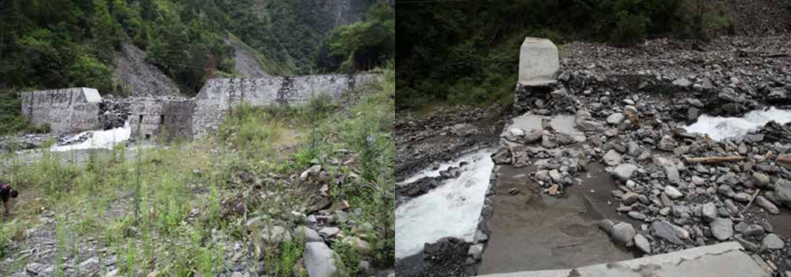
Figure 19: Weak civil structure as seen in Yikeying gully, Li county is not effective to contain large volume of debris
