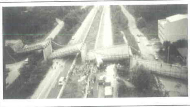
Figure 3.14. Collapse of Arifiye overpass on TEM highway (Erdik, 2003)
