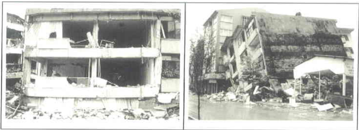
Figure 3.11. Strong beams weak columns (Bruneau, 2002)
