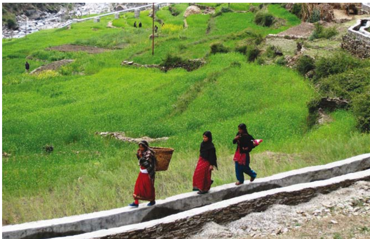
An irrigation channel in the Bhatakatija municipality of Far West Nepal, which also leads water to a 30 kW hydropower plant
