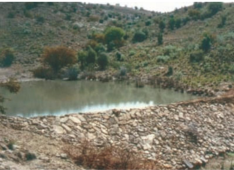
or 'zabo', are built on the ridge tops, and the middle terraces to collect runoff. The stored water is used for the animals, and then runs down to the paddy fields.
