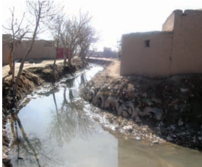
Irrigation canal near settlements in Injil district of Herat province. The community uses truck tires and plants trees to protect the houses from floods and to limit soil erosion
