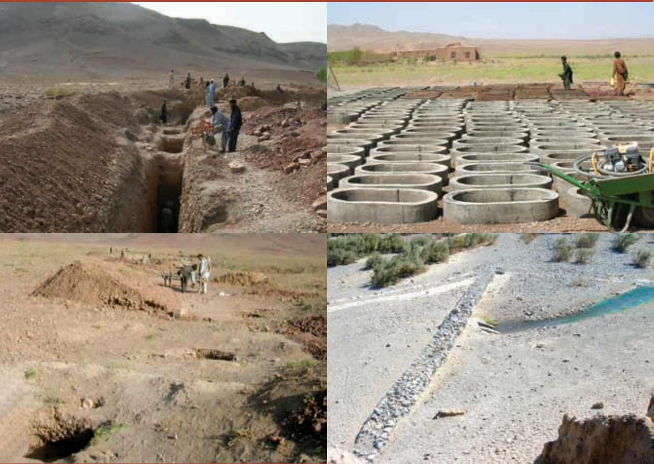
Figure 2: Kariz rehabilitation in Adraskan district, Herat: (a) Communities are digging a new channel for the Kariz irrigation system after it had been destroyed by floods; (b) Concrete rings to reinforce the tunnel; (c) Covering the tunnel with soil; and (d) A gabion wall protects a Kariz outlet in Sangi district, Herat
