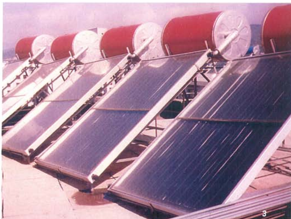
Solar water heater on the roof-top of an apartment building, China
