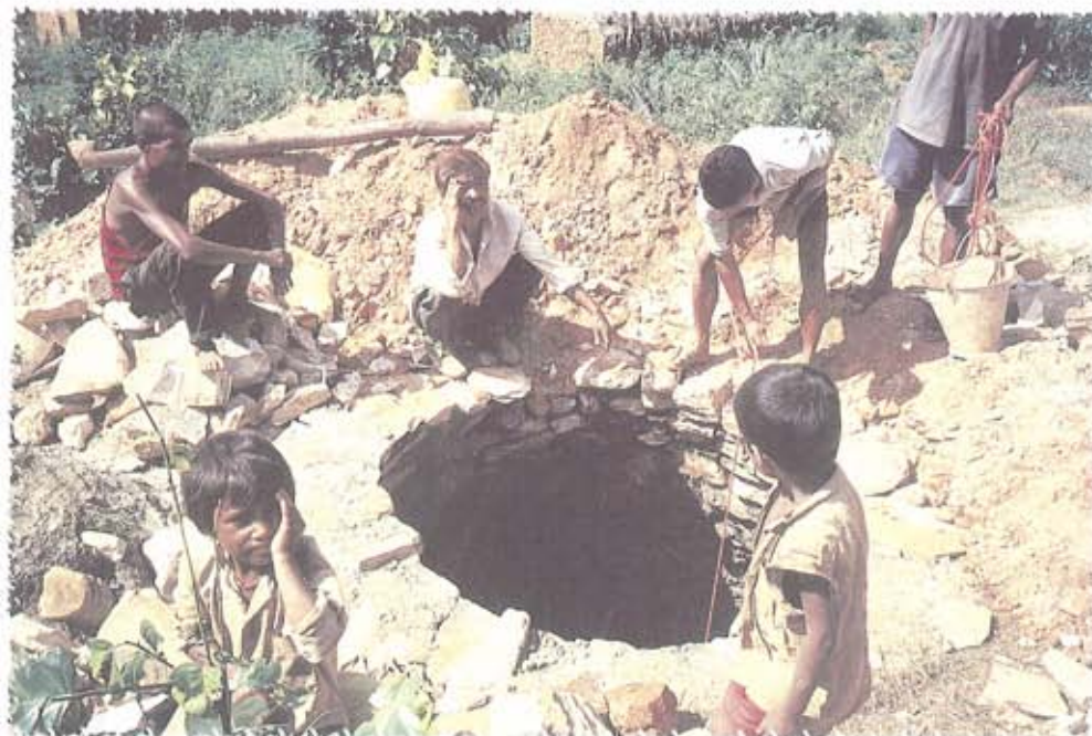
Construction of an underground water harvesting tank in the Jhikhu Khola watershed in Nepal
