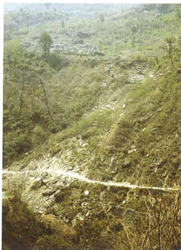
Plate 4: Landslide in shrub area, crossing road + deterioration of road supports
