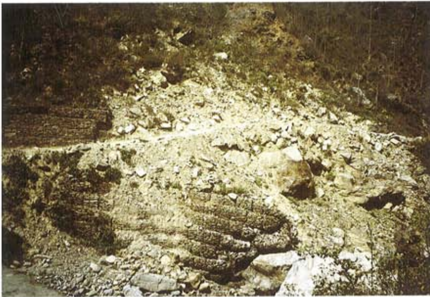
Plate 3: Landslide and Deterioration of Roadside/Supports
