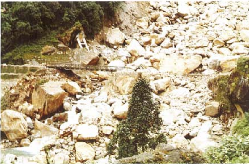
A new bridge constructed in the same location of the old bridge which was completely destroyed by debris flow in 2000 is still at risk (South Bhutan).
