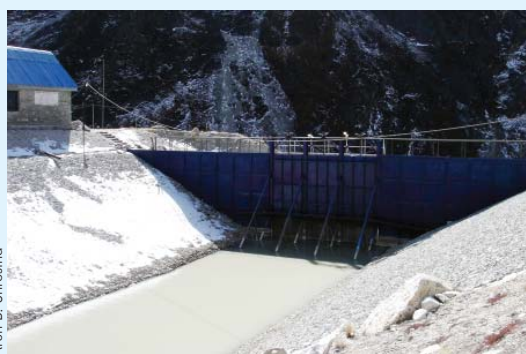
The gated open channel constructed in 2000 to lower the lake water levels
