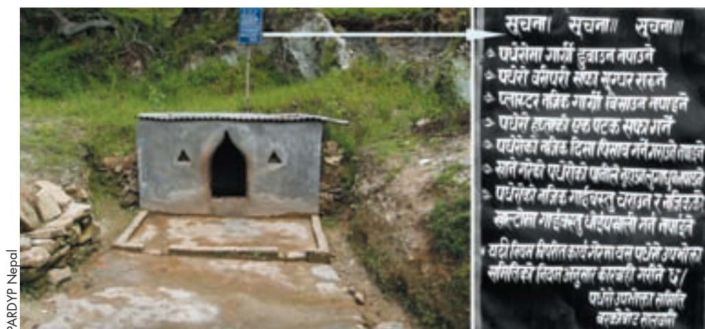
Figure 2: Community-based rehabilitation with rules for proper management of Dhotra springs in Nepal has led to increased drinking water security for spring users
