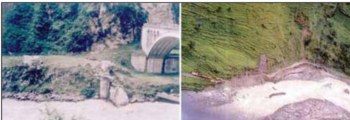
Figure 20: Remnants of a bridge pier (left) on the Arniko Highway and a section of the highway destroyed by the 1981 Zhanzangbo GLOF
