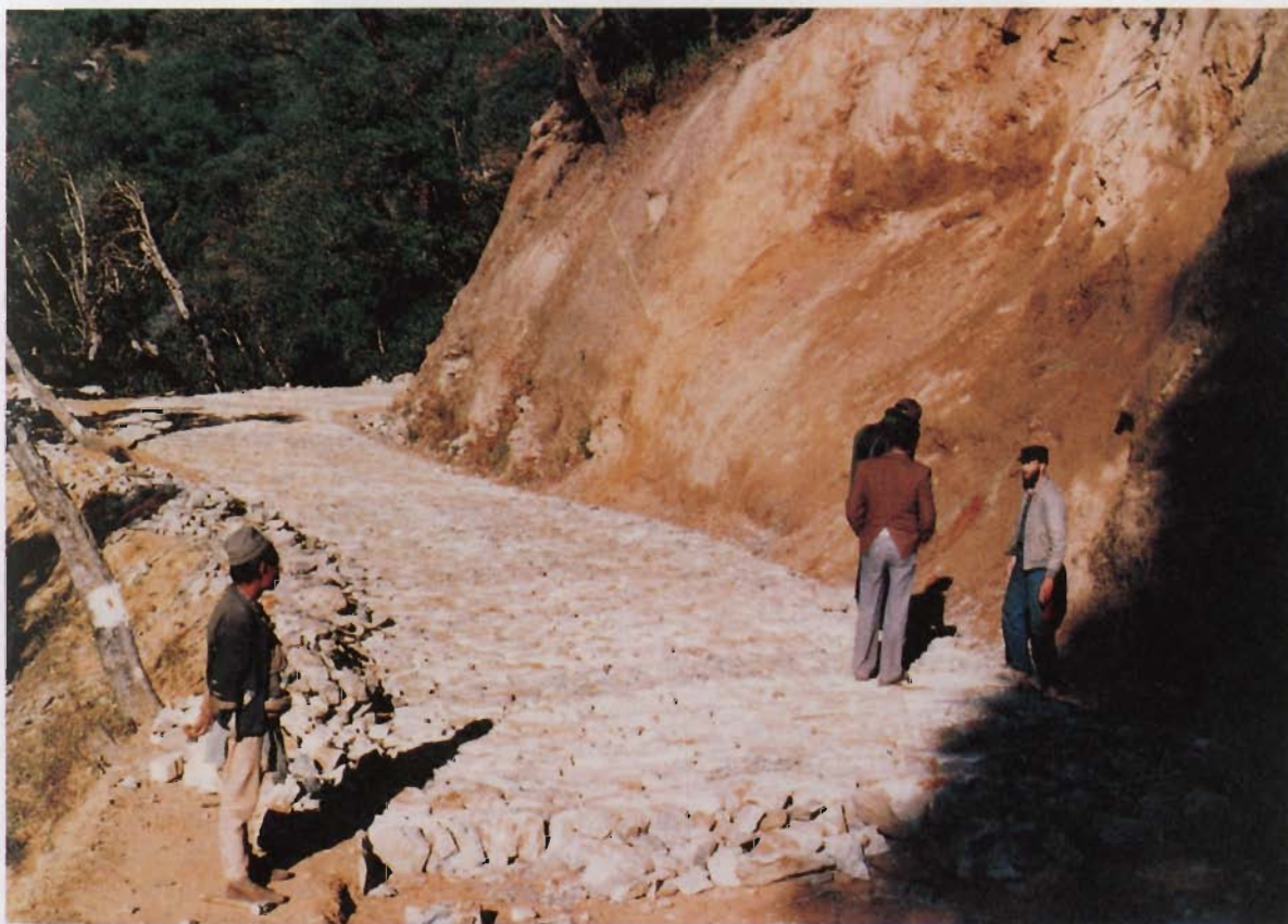
Plate 5: 20 cm thick stone soling layer on the subgrade.
