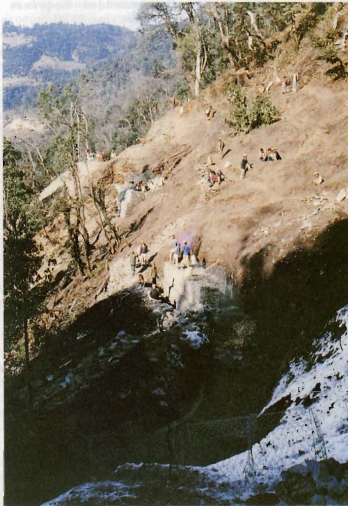
Plate 27: Erection of vs walls before the excavation of the road profile starts.
