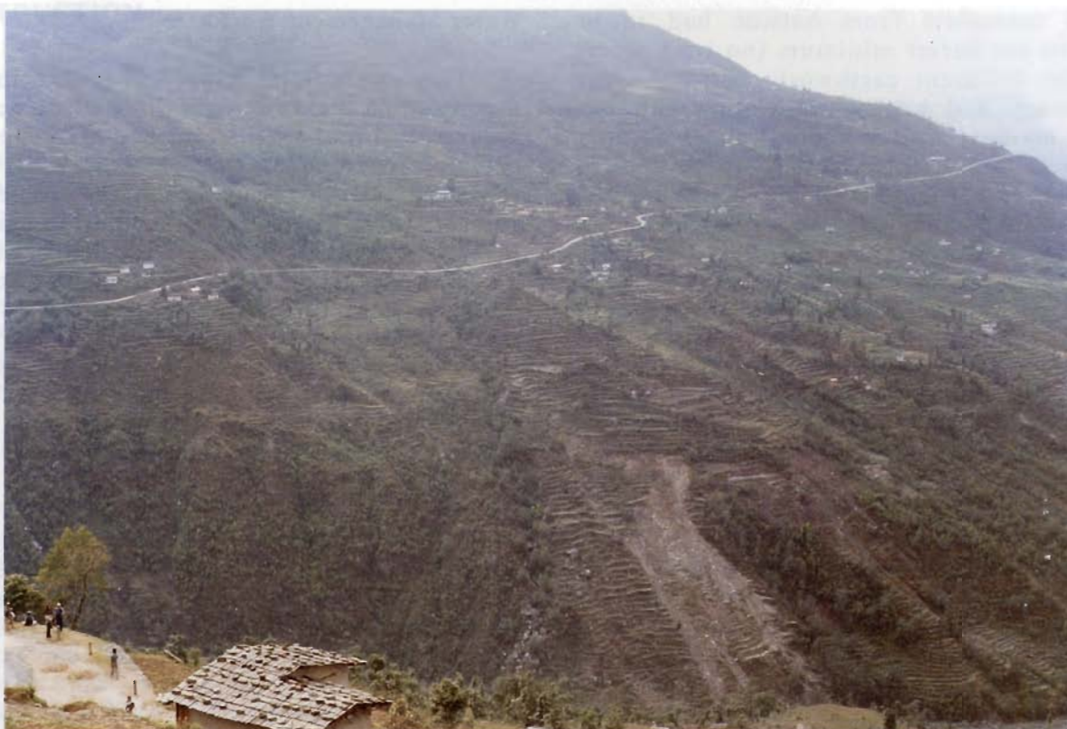
Plate 14: The mass balance has been achieved. The road is hardly visible and its vicinity intact.
