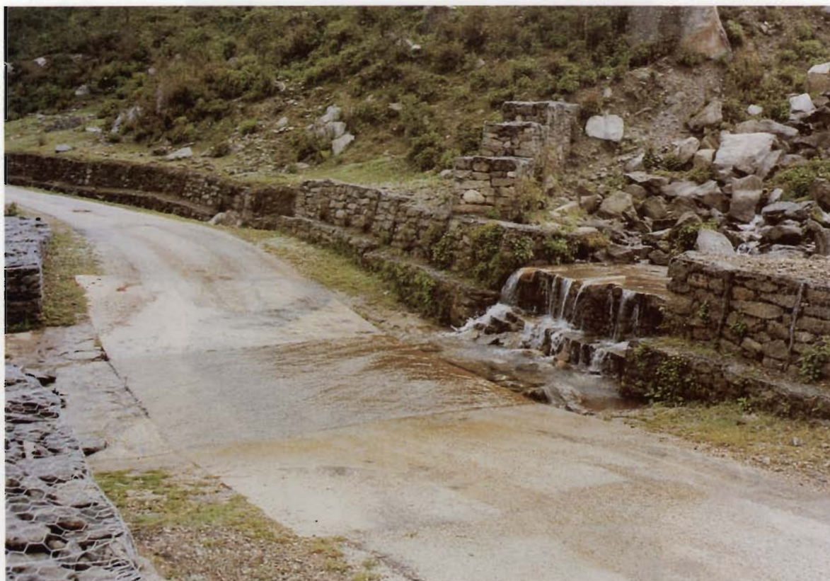
Plate 18: Causeway with water guiding inlet and outlet structures.
