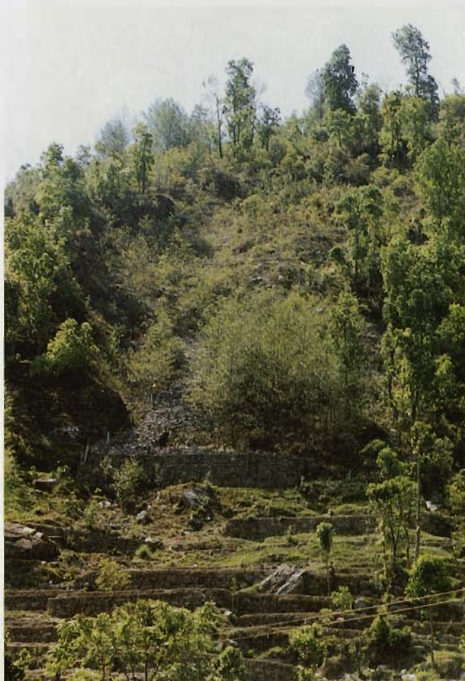
Plate 25: Again, a slide protection with structures consisting of a footwall with stone layer above and systems of stone arches (not visible) combined with planting of vegetation (3 years after construction).
