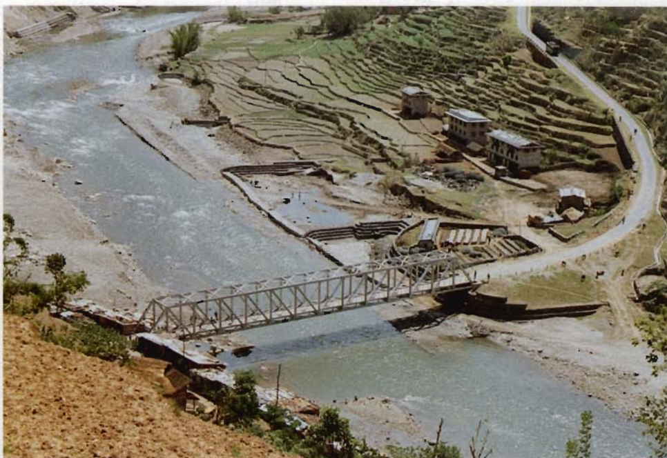
Plate 20: Sun Kosi Bridge. The erosion protection structure above the bridge consists of 4 spurs on the right embankment and 5 spurs on the left side, of which only the 2 highest ones are still visible (the other ones are already covered by river gravel and have therefore fulfilled their task)
