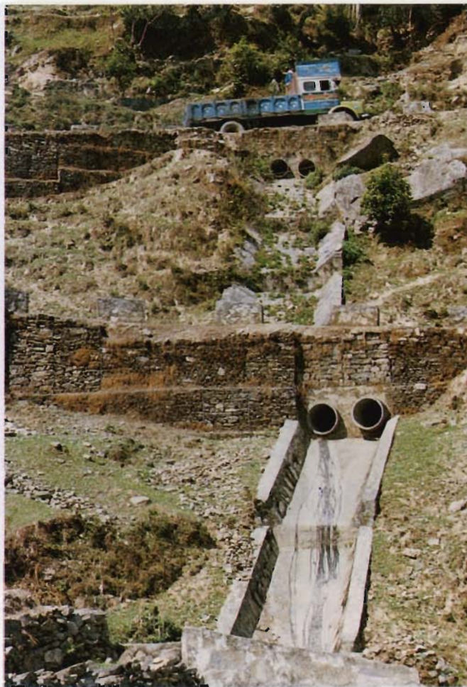
Plate 17: Two subsequent double pipe culverts 0.60 cm with controlled outlet over some distance.
