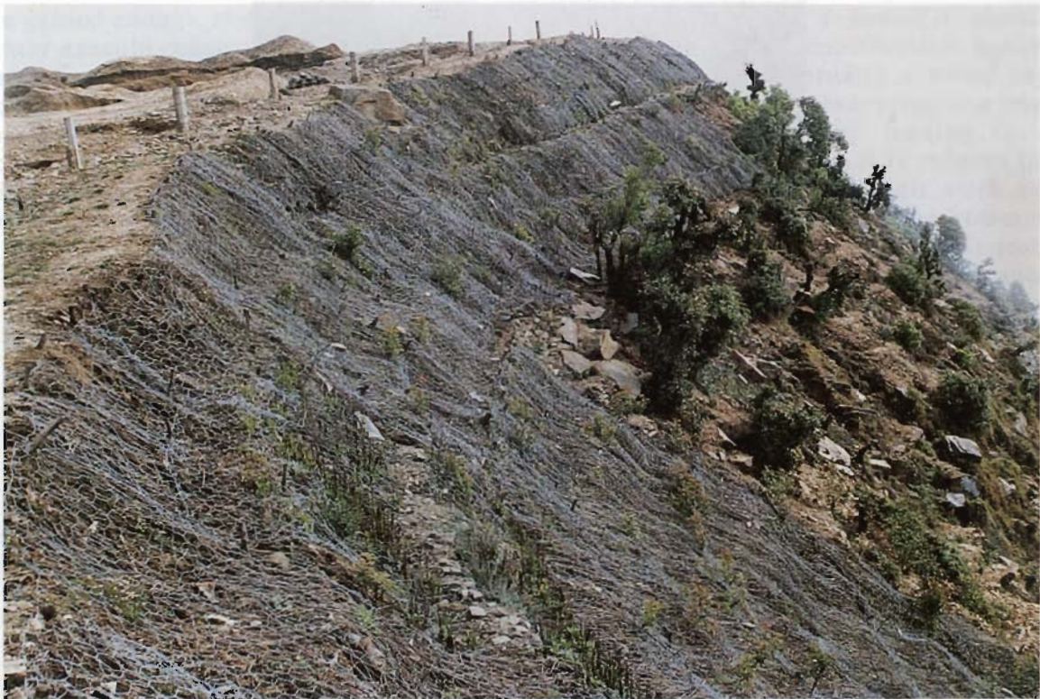
Plate 22: Same bioengineering technique, but covering the branches with wire netting instead of nailing them. This cover has to be dismantled after due time. The protected area is fenced off with barbed wire.
