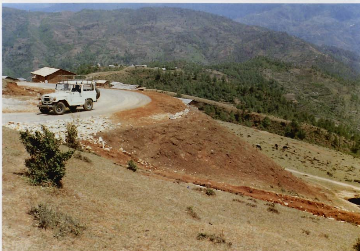
Plate 15: Embankment of more than 5 m height near Jiri. The surface is protected by the plantation of grass bunches.
