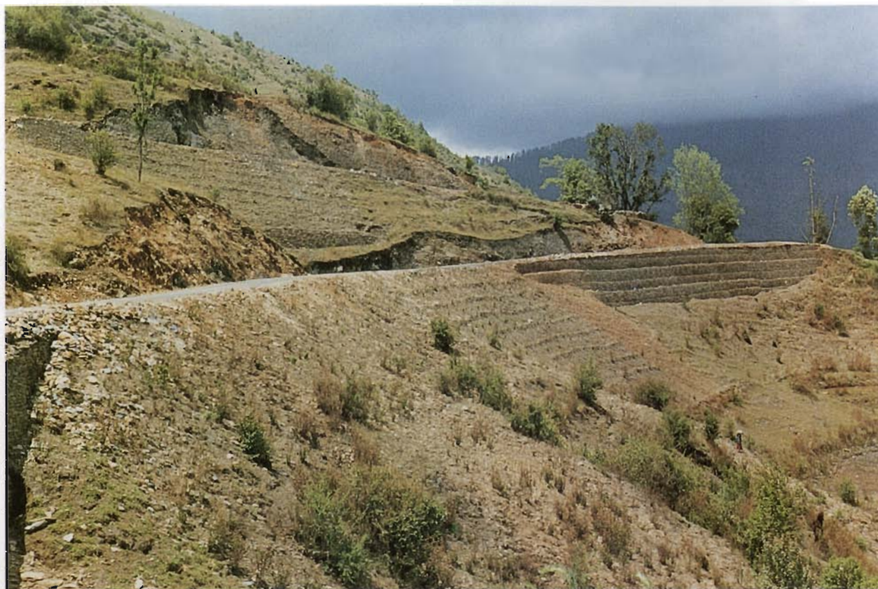
Plate 10: Cut and fill balance in the long section.
