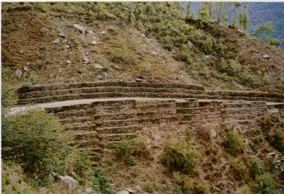
Plate 7: The slope of this road section is so steep that a retaining wall on the vs and a toewall on the ms were constructed.
