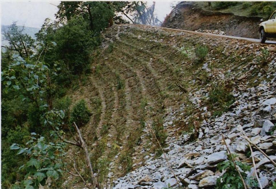
Plate 21: A vs slope surface protection by bioengineering: fast growing branches fixed on the slope by gabion wire and nailed with cutting sticks.
