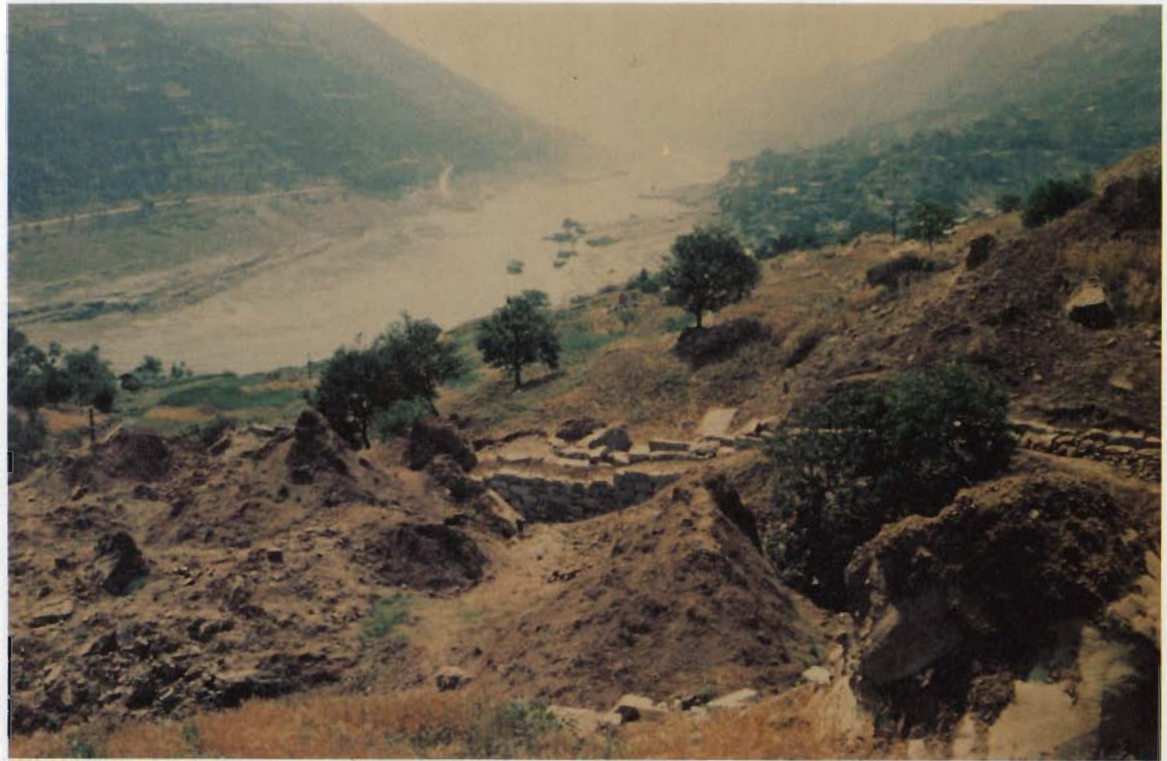
The landslide is shown in the foreground, the Changjiang River in the middle background, and the county site of Yangyang on the banks of the Changjiang River in the background - to the right. Courtesy of Wang Zhiru.
