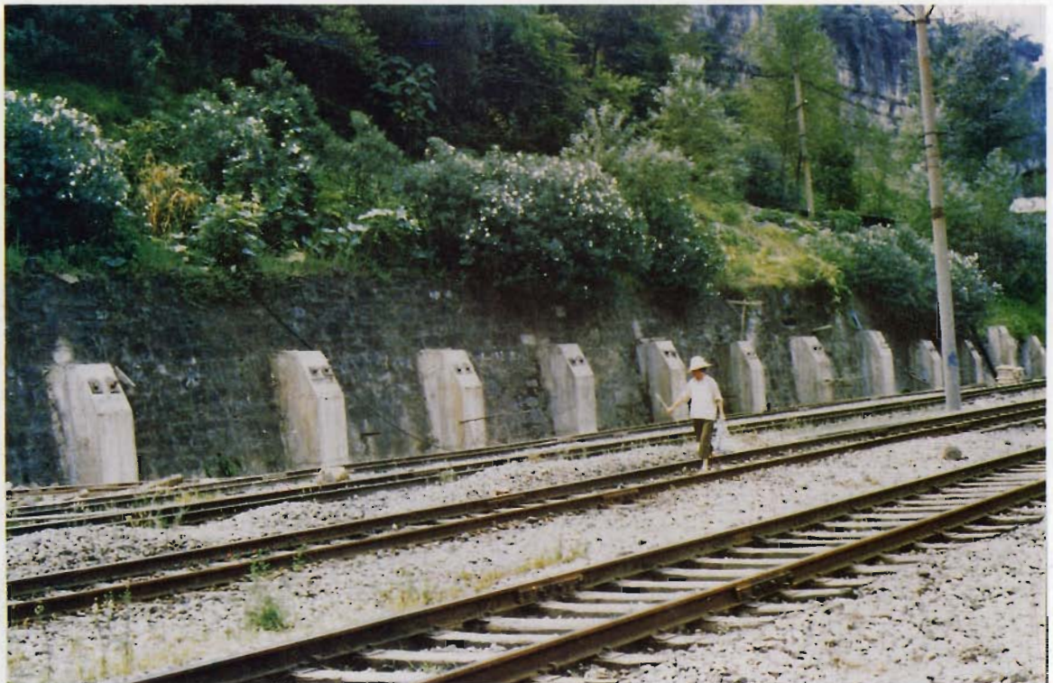
The use of anchor-rope driven piles (centre, background) to stabilise landslides
