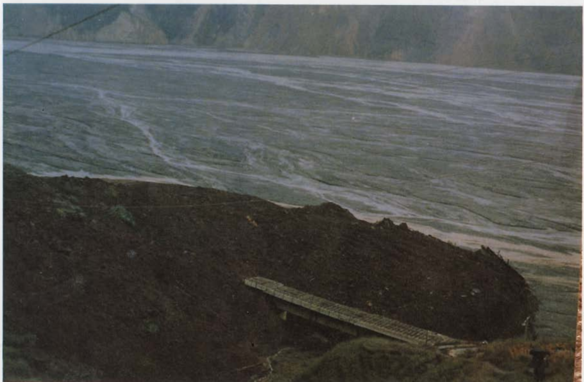
Plate 4 : Forward Movement of the Railway Embankment by 100m and Destruction of Two Railway Bridges at Dalisu in Dongchuan District (Oct. 6, 1986)
