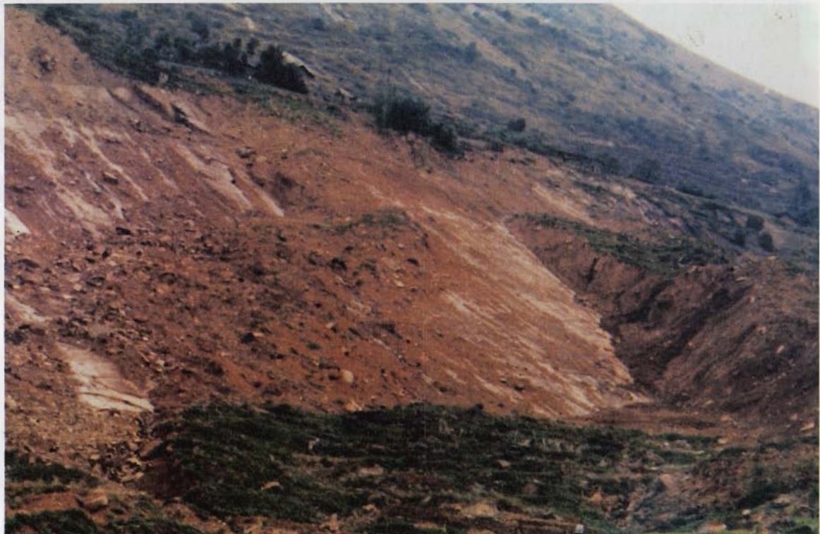
Plate 6: A Close View of the Upper Section of the Jipazi Landslide (Looking Northwards)
