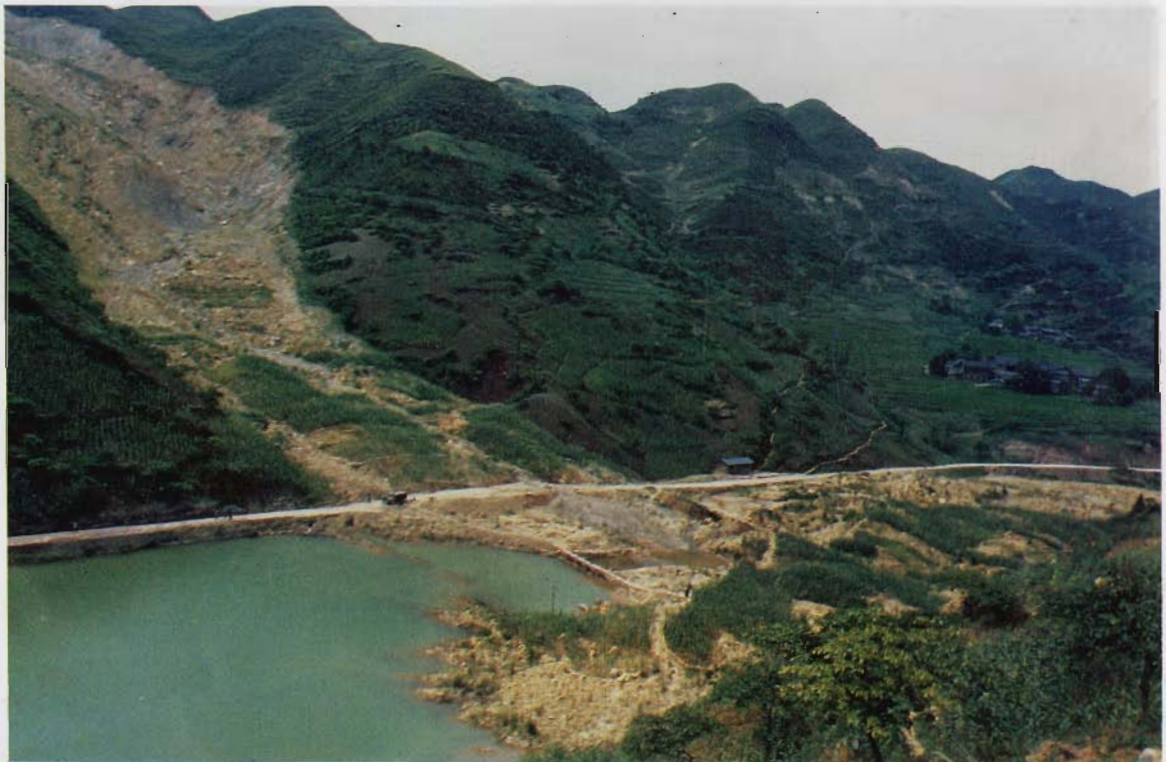
The landslide dam formed in July 1982 during heavy rainstorms in Eastern Sichuan. This photograph shows the lake (foreground), remains of the Geling landslide dam (foreground), and the landslide (background).
