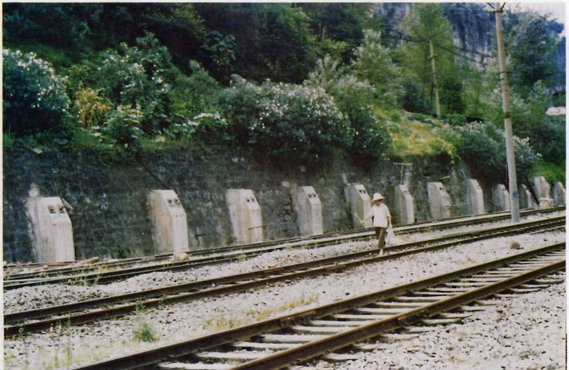
Plate 15: Control Works at the Jianjiyan Landslide, Songzao Coal Mining Area, Sichuan Province
