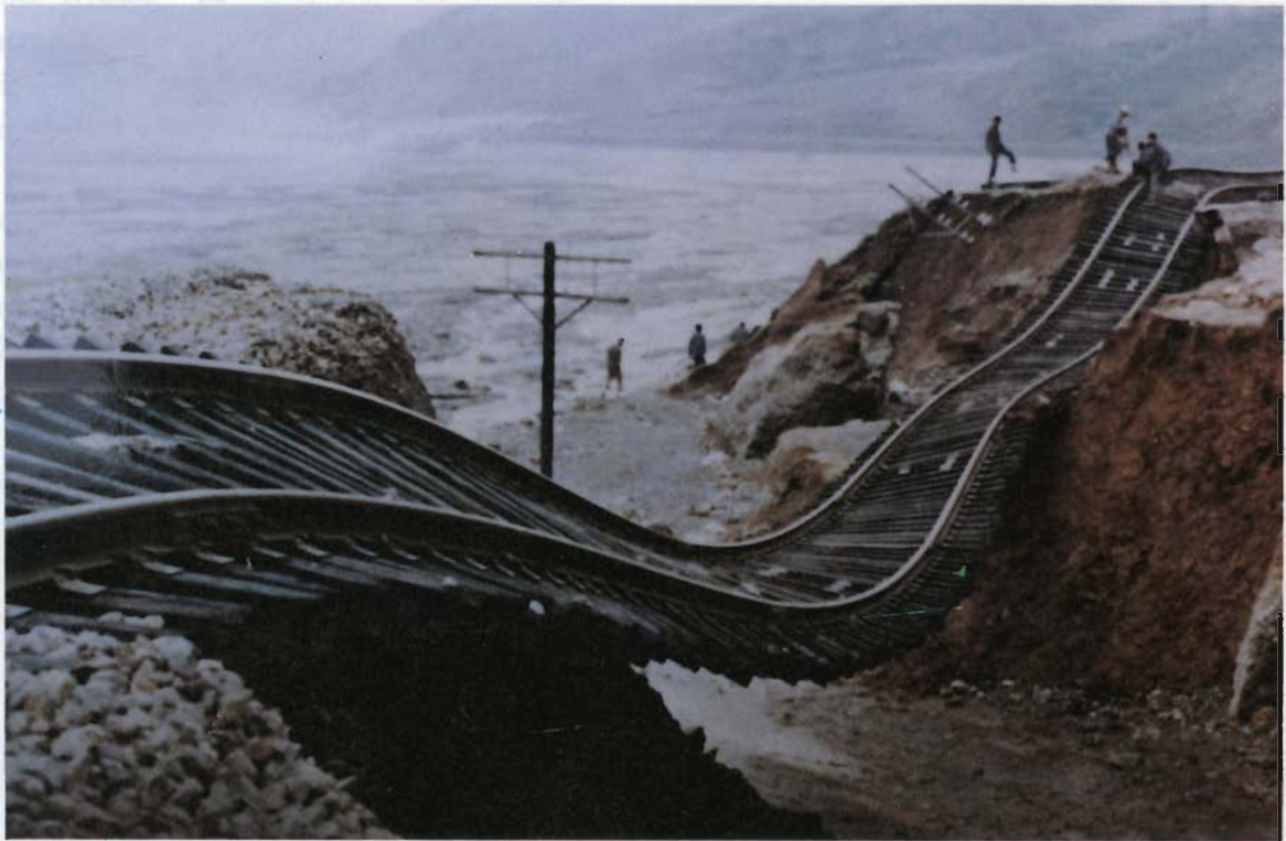
Plate 3: Debris Flow Undermining the Embankment of Dongchuan-Kunming Railway (1 July, 1985)
