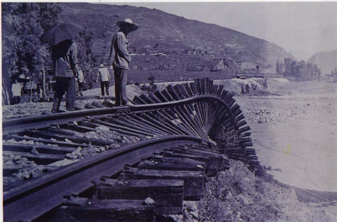
The embankment was undermined by debris flow and flooding following breaching of a debris flow dam formed on 30 June, 1981. Courtesy of Yang Wenke
