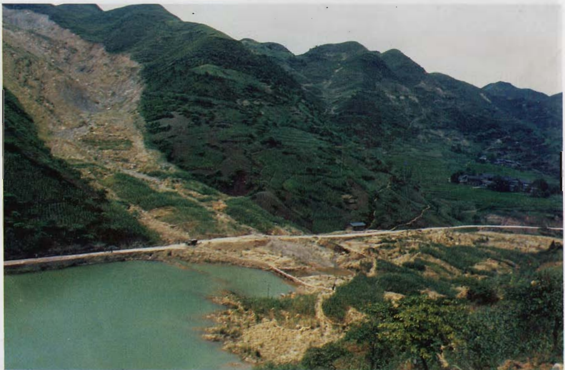
The landslide dam formed in July 1982 during heavy rainstorms in Eastern Sichuan. This photograph shows the lake (foreground), remains of the Geling landslide dam (foreground), and the landslide (background).
