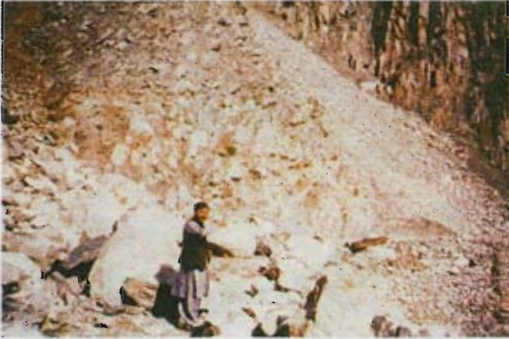
Landslide across road
