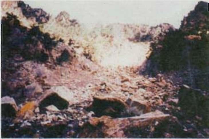
Erosion above road
