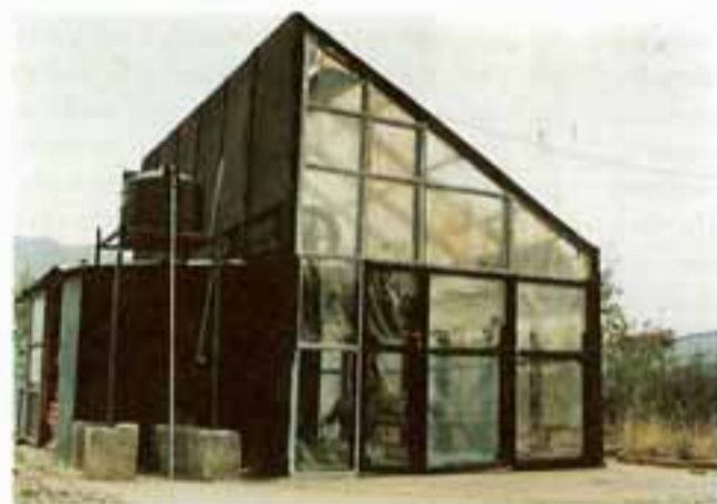
Low-cost Solar - Timber Kiln Installed at Energy Park, Dr. Y.S. Parmar University of Horticulture and Forestry, Solan, H.P., India
