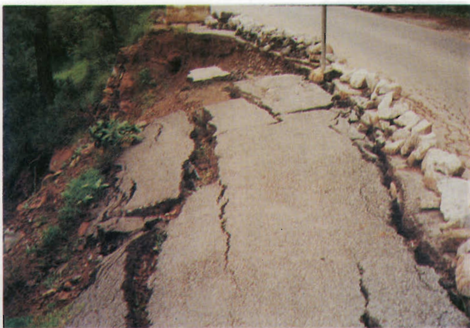
Plate 7: Subsidence of metalled road near Kohala
