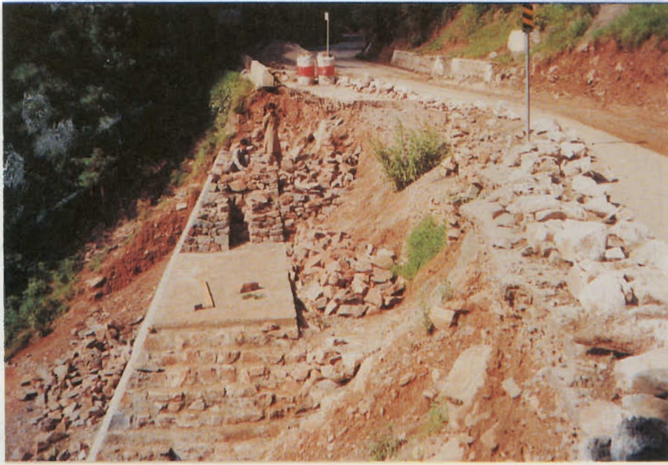
Plate 5: Reconstruction of retaining wall after landsliding along the Murree-Muzaffarabad Road
