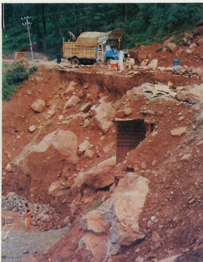
Plate 4: Failure of retaining wall due to slump failure
