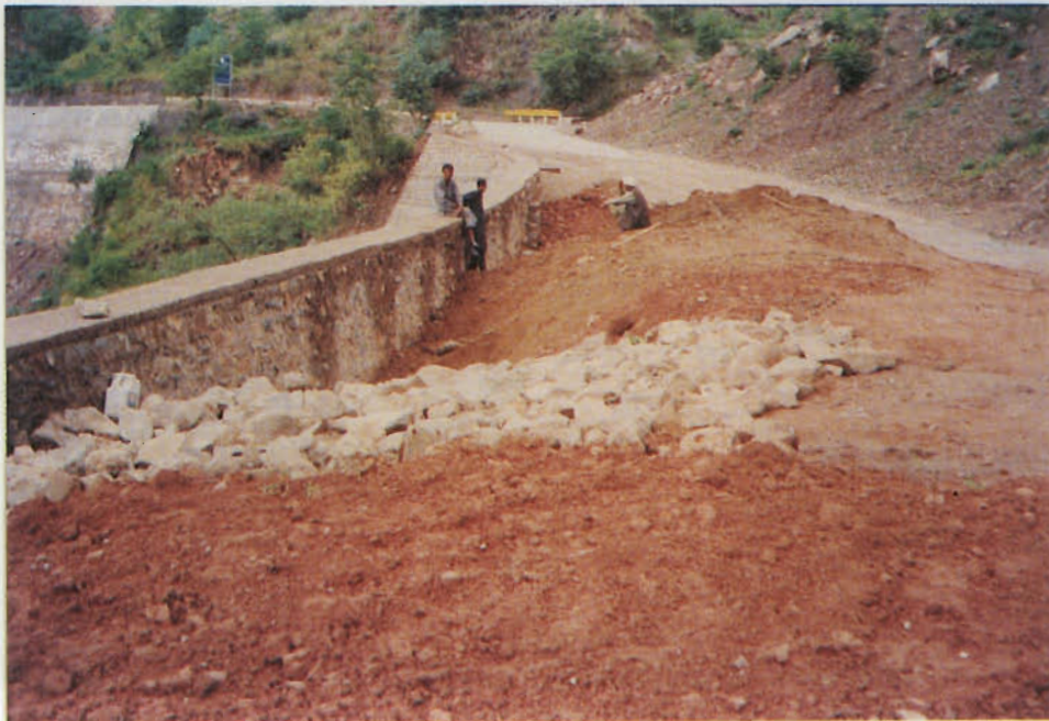
Plate 6: Backfilling behind the retaining wall along the Murree-Muzaffarabad Road
