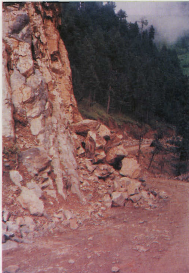
Plate 14: Widening of road by blasting (may cause threatening slope ultimately)
