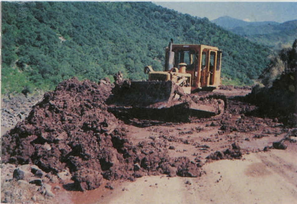
Plate 2: Landslide between Muzaffarabad and Garhi Dupatta (Failure is within the ancient landslide)
