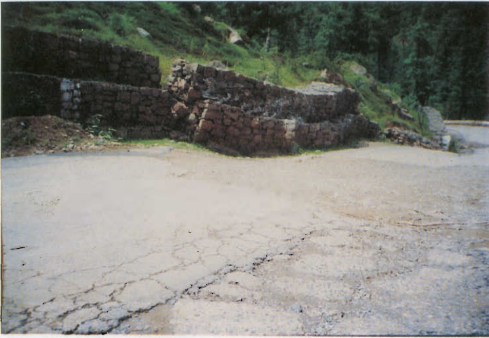
Plate 1: Medium-sized gabion structure showing deformation due to creep
