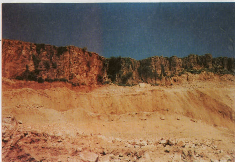
Plate 18: Fresh slip surface (Aug. 1994) along the M1 Motorway (Simbal landslide) between Lahore and Islamabad
