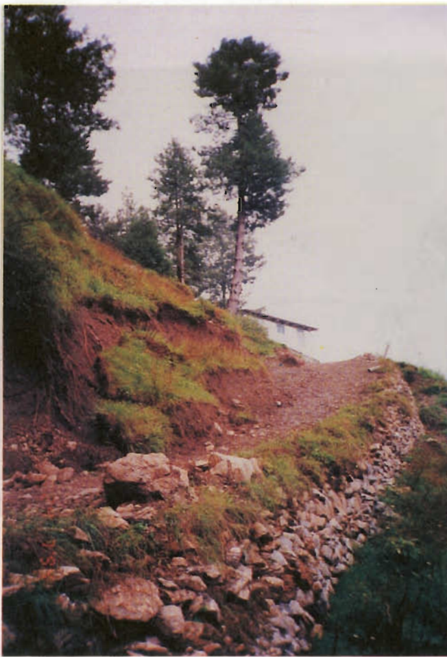
Plate 13: Small-scale landslide caused by making a path for a newly-built house
