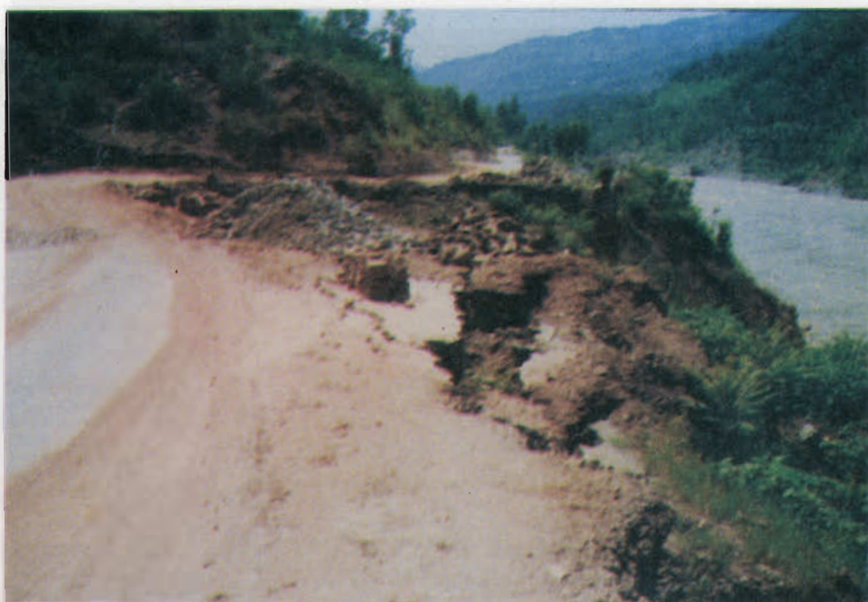
Plate 8: Initiation of failure of downslope due to absence of retaining wall
