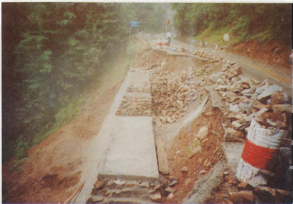
Plate 3: Downslope failure of the retaining wall due to landslide as a result of saturation
