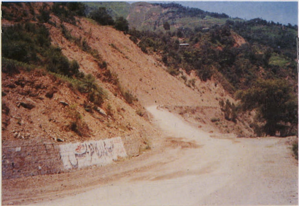
Plate 12: Movement of scree slope blocking the road between Muzaffarabad and Garhi Habib Ullah
