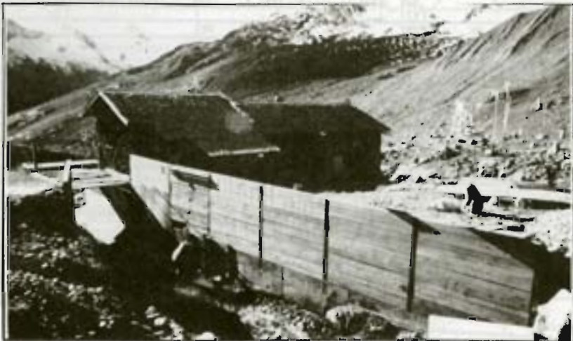
Figure 6: Structural Changes in the Upstream Section of the Vernagtbach Gauging Station to Increase Throughflow Capacity. Upper Photograph (30 June 1993): The Original Situation; Lower Photograph (8 Oct. 1995): After the Construction of Wooden Wall with a Concrete Lower Section
