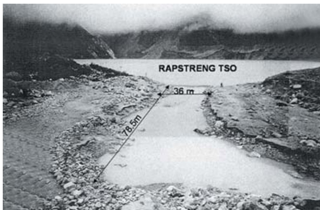
Figure 6.20: Raphstreng Tso outlet expanded by manually digging through the end moraine in 1998, see Figure 2.9 for location
