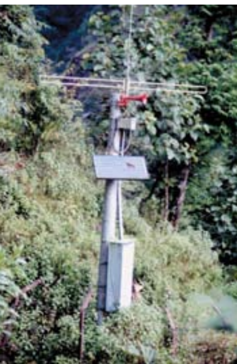
Figure 6.2: Early warning system installed at Gongar village. The systems consist of a solar panel, battery, antenna and amplifier with siren.
