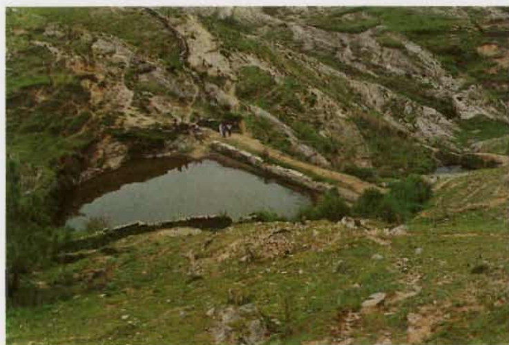
Plate 2: Rain water-harvesting pond built through the 'Self help' programme by the villagers of 'Kandi Bagri' with a provision to collect the seepage flow in another pit at the lower end
