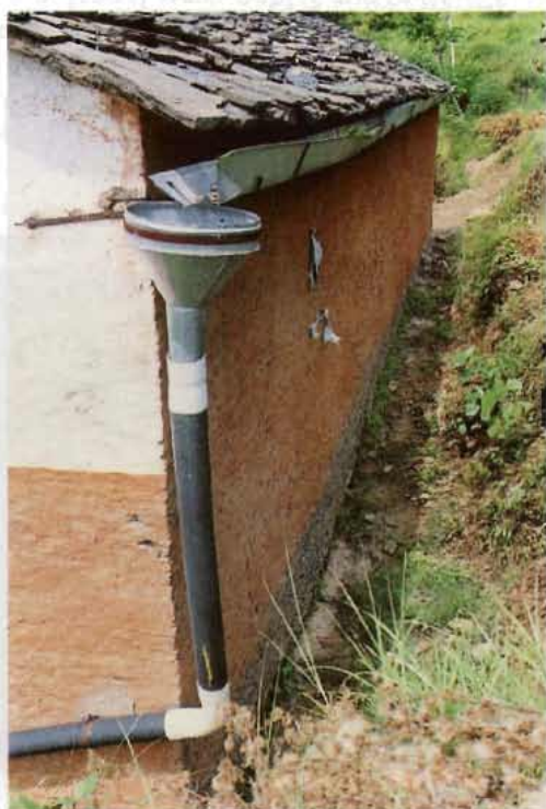
Plate 3: Roof-water harvesting being practised by the farmers in a traditional way from the slanting slated roof of a house
