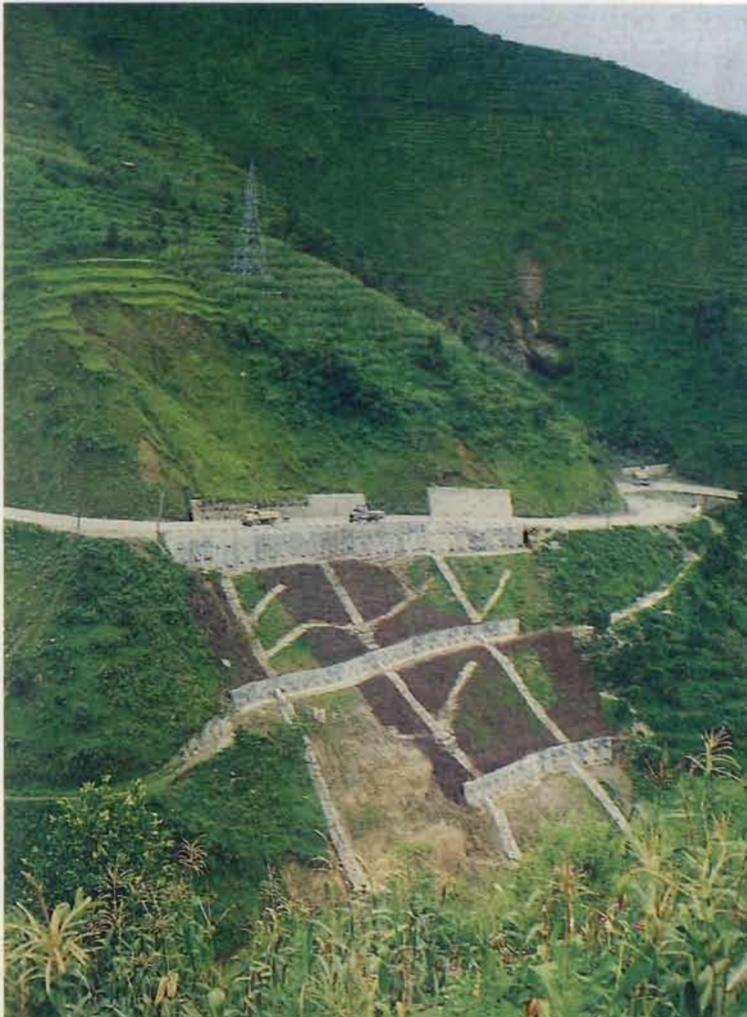
**Plate 10:** Landslide stabilisation measures (retaining walls, rock anchoring, surface and subsurface drains, and bioengineering works) applied at the Khatripauwa Landslide along the Thankot-Naubise road, Central Nepal - view towards the southwest.
