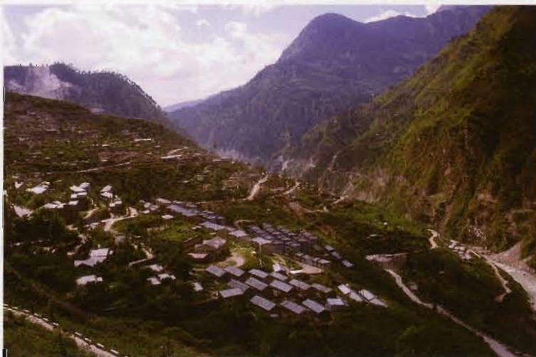
A new road, hydroelectric plants and incipient industry have created a mini-urban corridor along a section of the Sutlej River in Himachal Pradesh.
