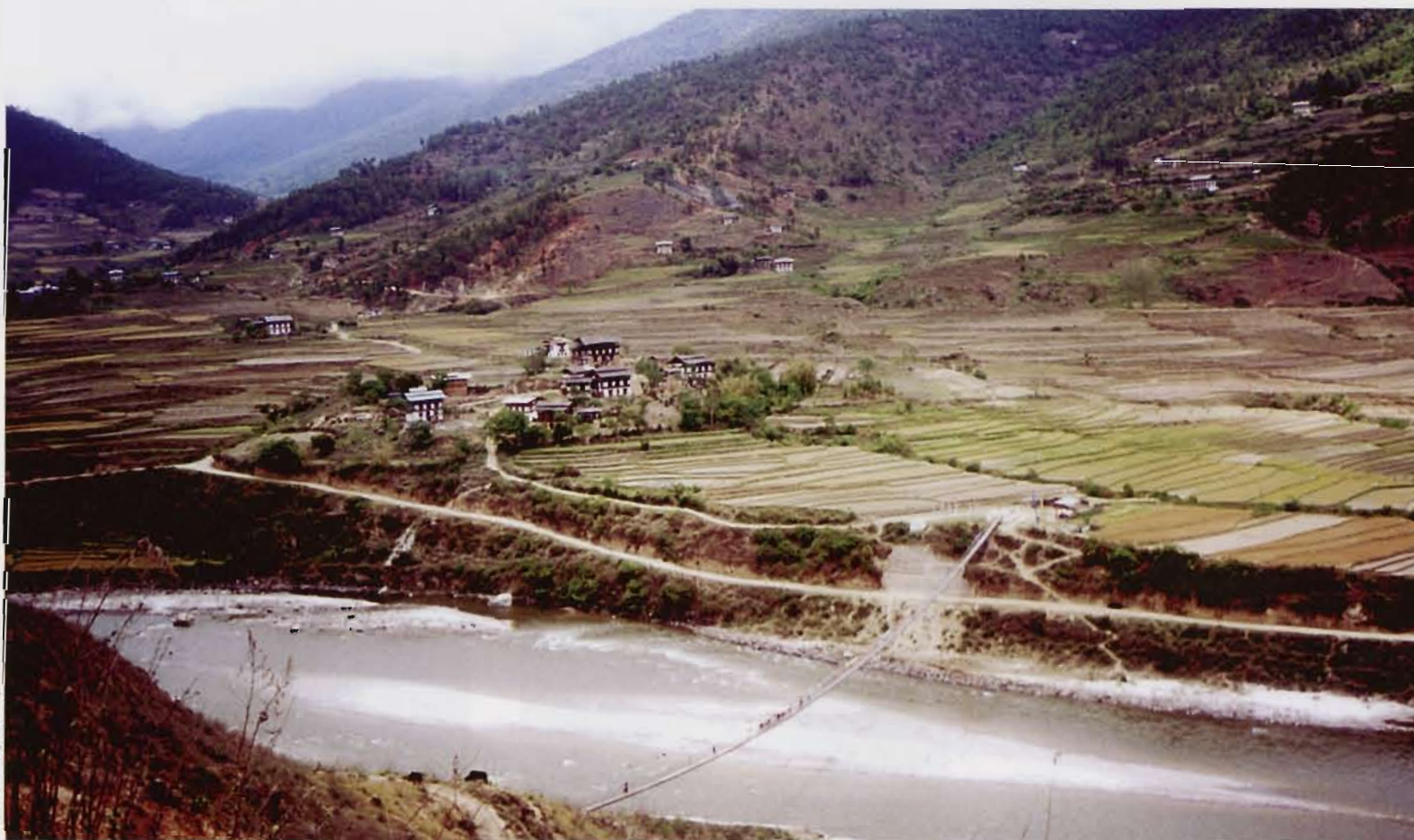
One of the longest suspension bridges in Bhutan over the Phochu river, Punakha.
