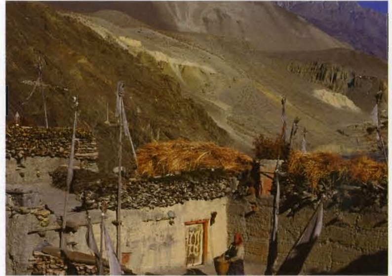
A flat-roofed adobe is common among houses in Tibetan-dominated villages of the arid, trans-Himalaya zone.
