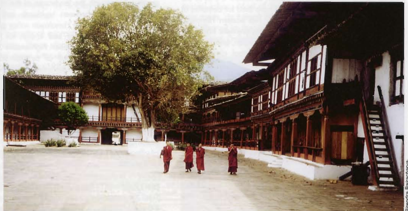
Wangdue Dzong, Wangdue, Bhutan
