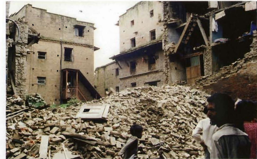
21 August 1988 earthquake, Bhaktapur, Nepal
