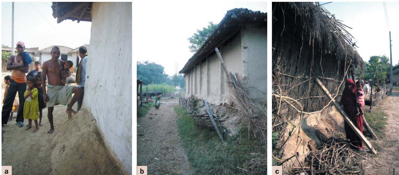
Figure 9: Strengthening and protecting walls and wall foundations: a) foundations protected with piled up mud, Katarait VDC, Dhanusha District; b) foundations protected with a bamboo fence and mud, Katarait VDC, Dhanusha District; c) wall made of bamboo, mud, and dried pulse plants supported by a wooden beam, Seurai VDC, Dhanusha District
