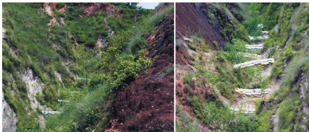
Figure 39: Bio-engineering activities for gully treatment
