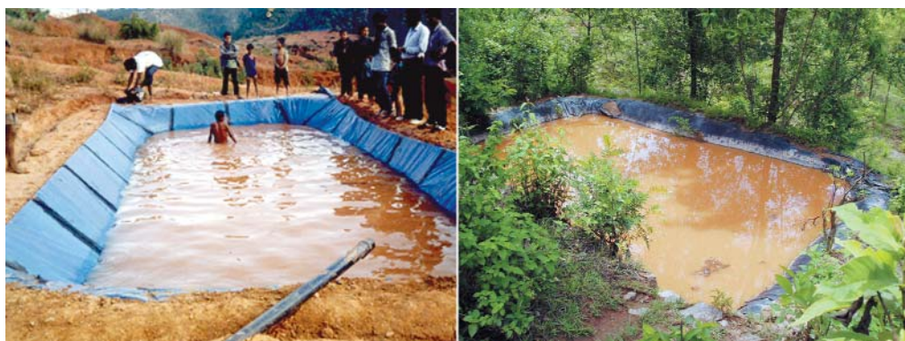
Figure 22: Plastic lined conservation ponds
