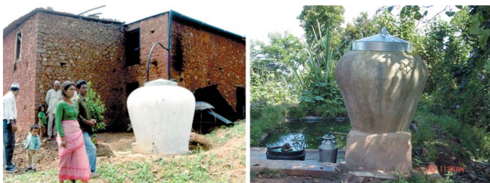
Figure 24: Roof-water harvesting system
