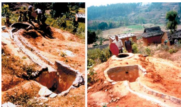
Figure 23: Underground water storage system
