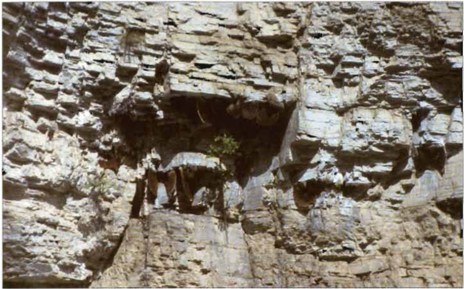
Listi Mai cliff next to the Nepal - China Highway: a large number of combs can be seen hanging under protruding rocks
