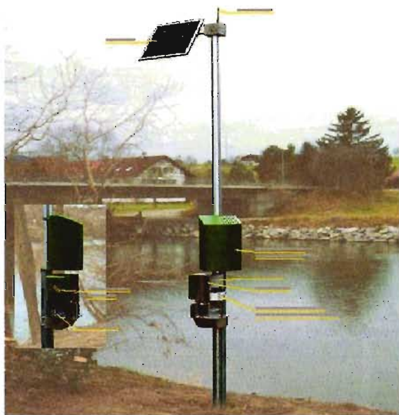
Figure 6: A fully equipped stand-alone hydrological measurement station (Source: OTT MESSTECHNIK, Germany)
