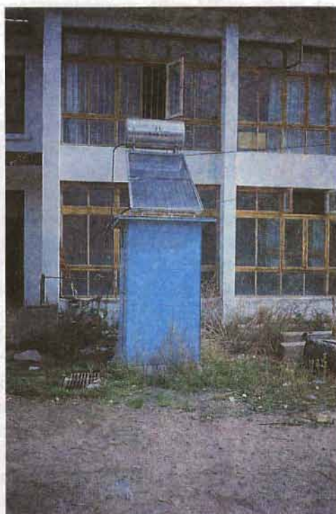
Solar water collector fitted on the roof of a bathroom, Lhasa, China
