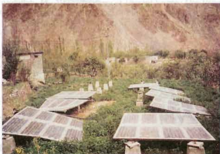
Plight of solar photovoltaic electrification scheme (30kW) due to lack of maintenance in the Northern Areas of Pakistan
