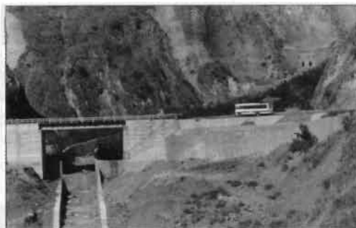
Figure 18.23: New bridge built in 1994 across the Laogan Ravine, the diversion flume can be seen under the bridge
