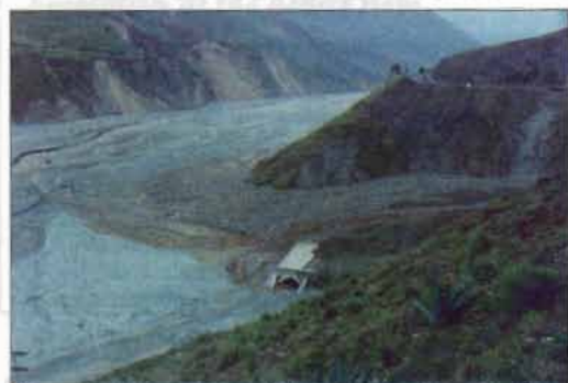
Figure 18.16: View of the covered tunnel and fan of the Laogan Ravine. The left outlet of the tunnel was silted up by about 3m as a result of the July 1987 flood
