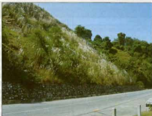
Plate 10.2: A steep cut slope in a weak sand deposit on the Naubise-Mugling road (central Nepal), stabilised with jute netting and grass planting
