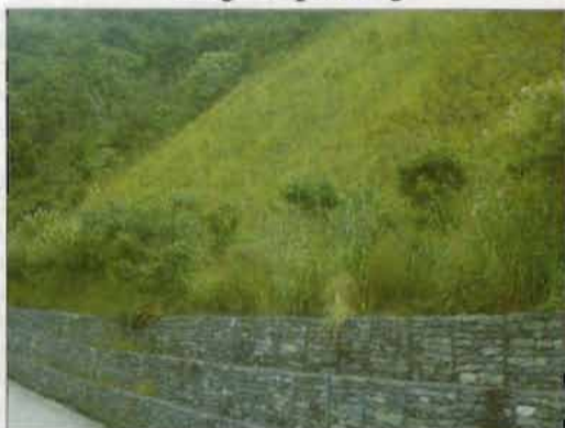
Plate 10.3: A typical cut slope in deep colluvium on the Dharan-Dhankuta road (eastern Nepal), stabilised using a combination of a gabion toe wall and bio-engineering
