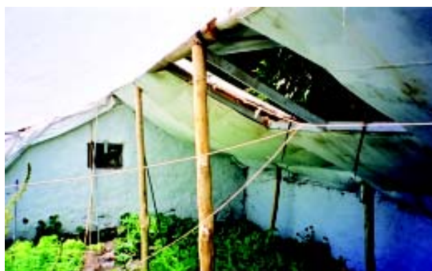
Figure 63: A white cloth added under the roof
