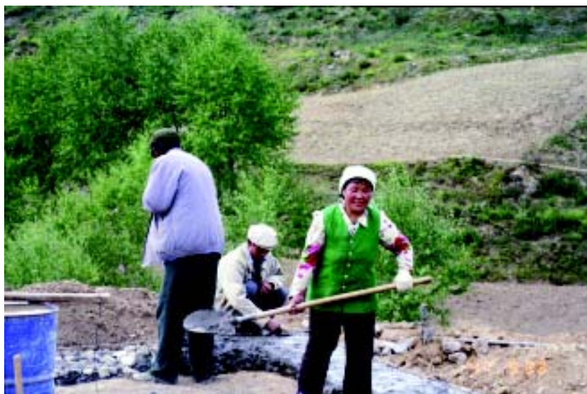
Figure 32: Covering the top of the foundation with a layer of concrete
