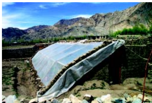
Figure 77: General view of fixing of the polythene sheet
