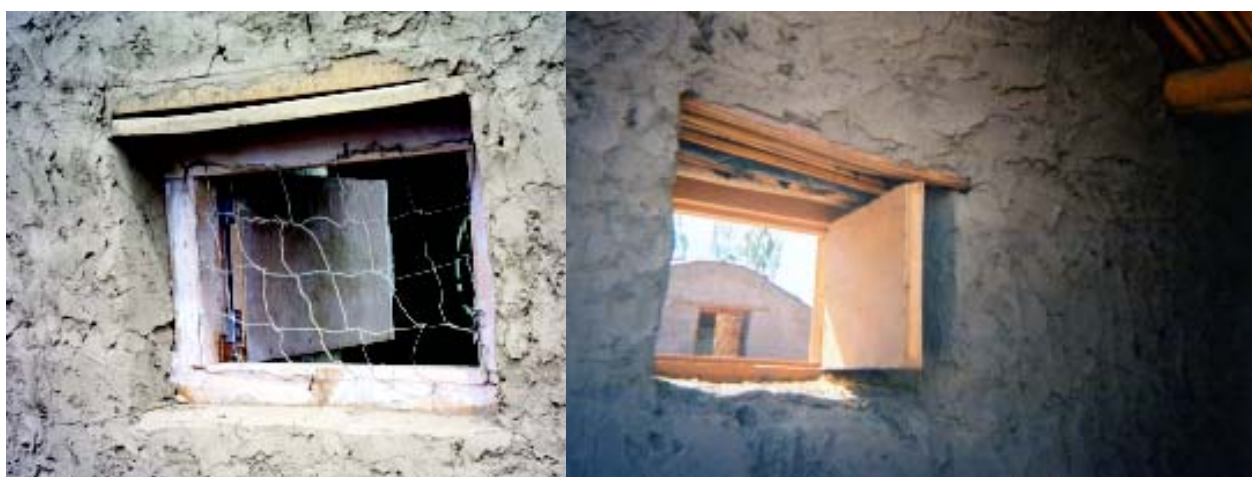
Figures 53 & 54: Inside and outside views of installed side shutter with chicken mesh outside
