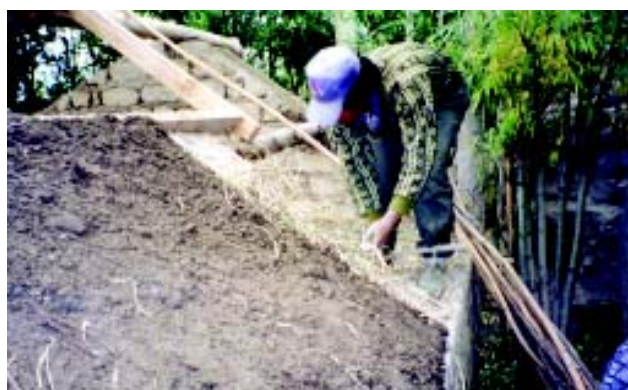
Figure 62: Applying the layers of cardboard, straw, and mud
