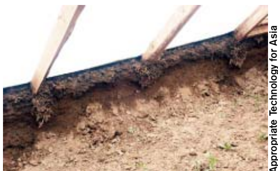
Figure 75: Joists balanced on a crumbling earth layer (outside ground level) in a greenhouse without southern foundations
