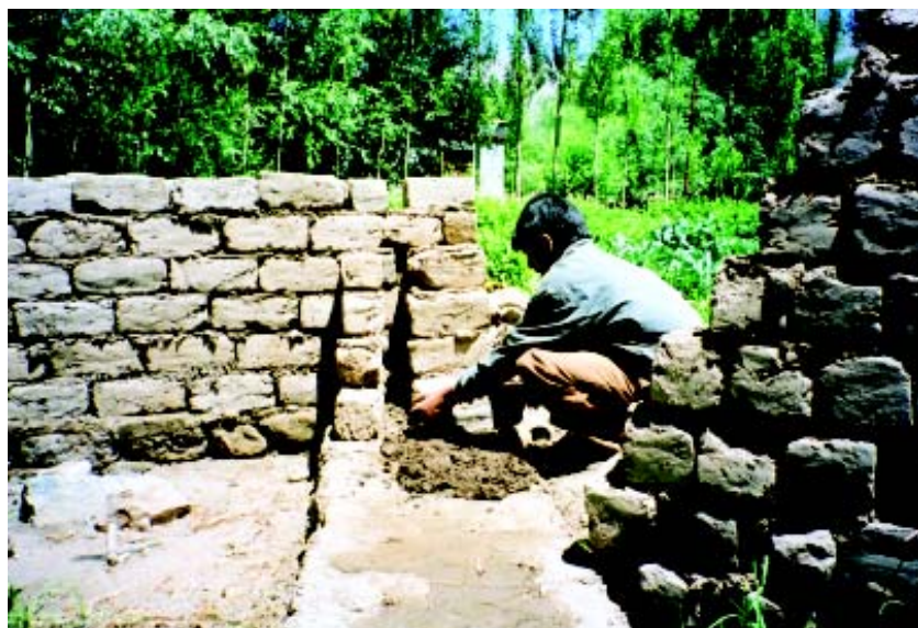
Figure 36: Building a double wall with mud bricks in Ladakh
