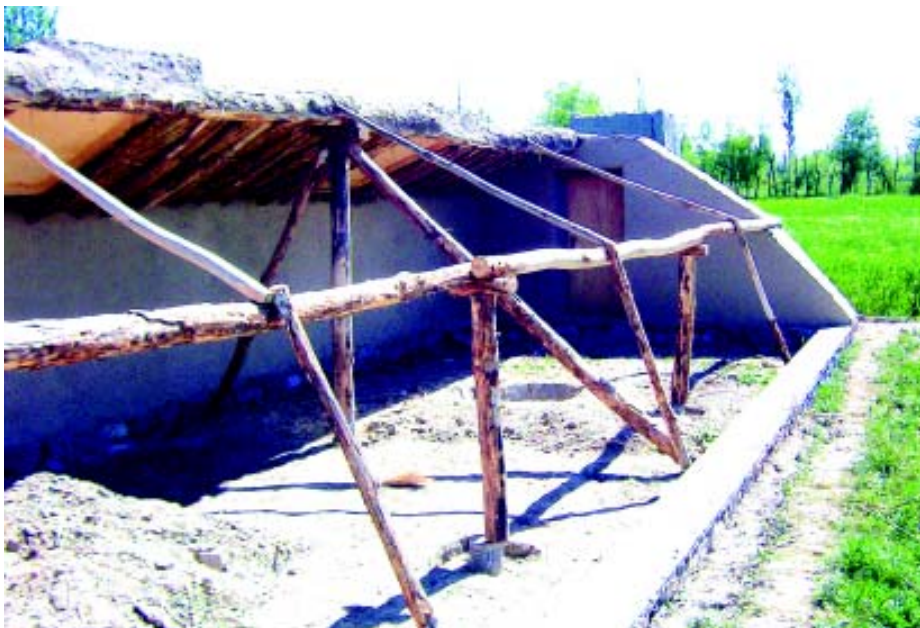
Figure 74: Wooden support structure for the polythene sheet (Lowgar, Afghanistan)
