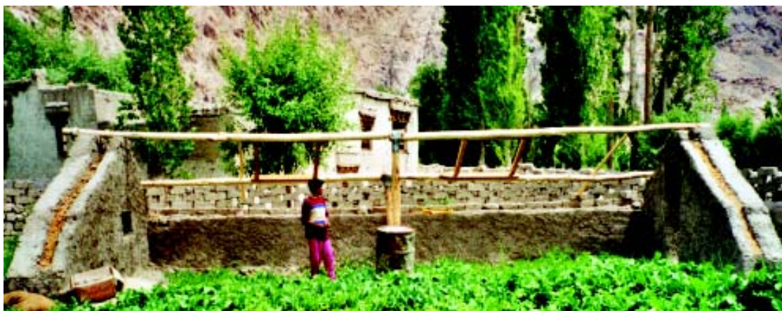
Figure 57: Roof structure with two beams and shutter frames in position in Spiti
