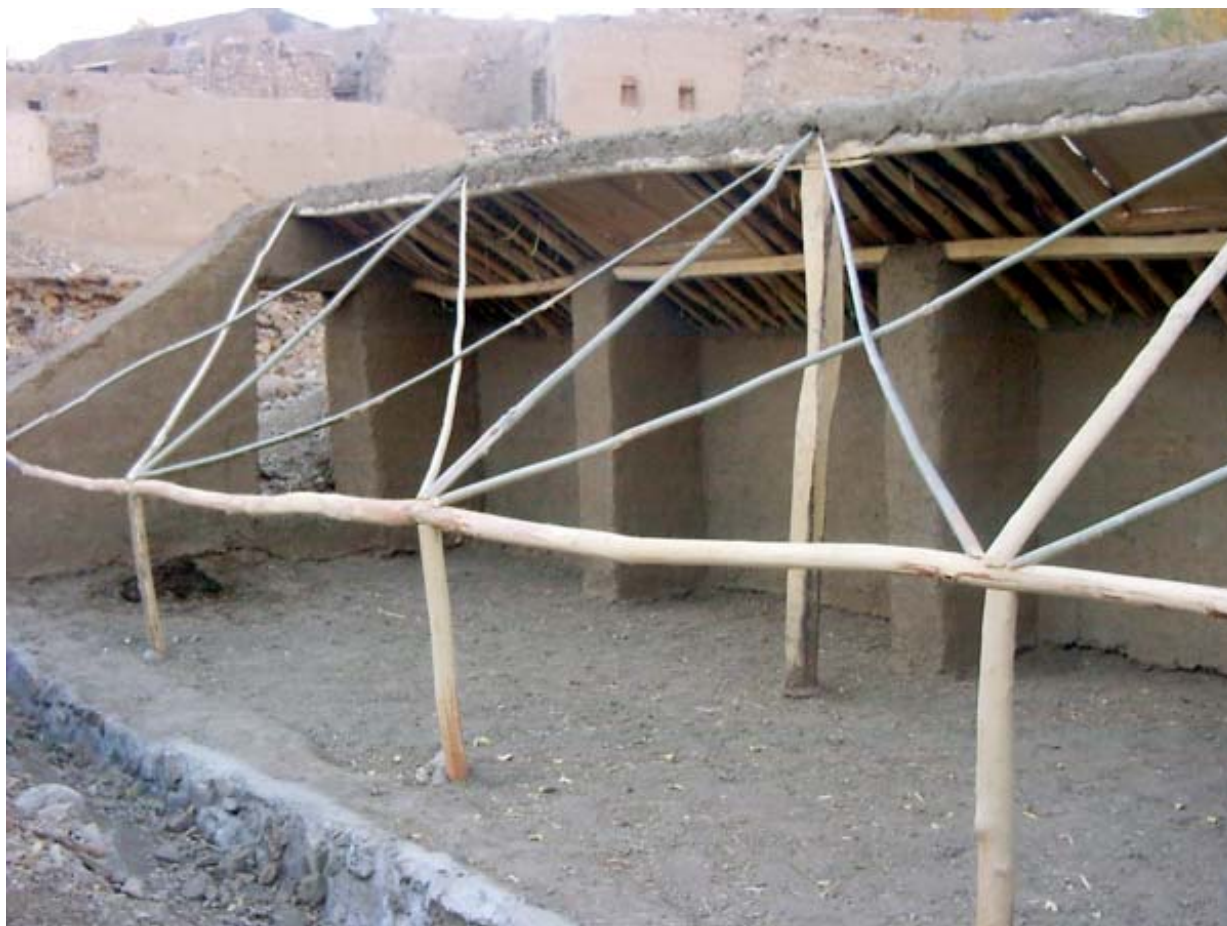
Figure 42: Completed inner partition walls, greenhouse in Zeback district, Afghanistan
