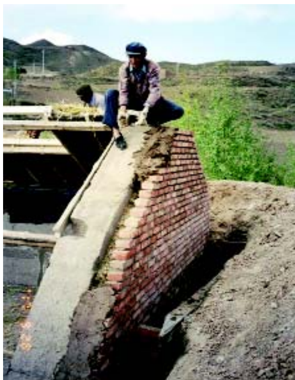
Figure 39: Construction of an outer wall with baked bricks and an inner wall with stabilised rammed earth in Qinghai
