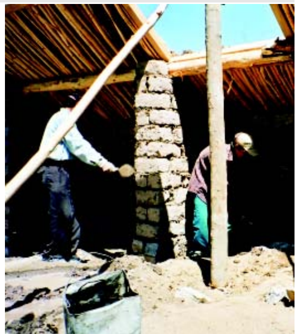
Figure 41: Finishing off the partition walls
