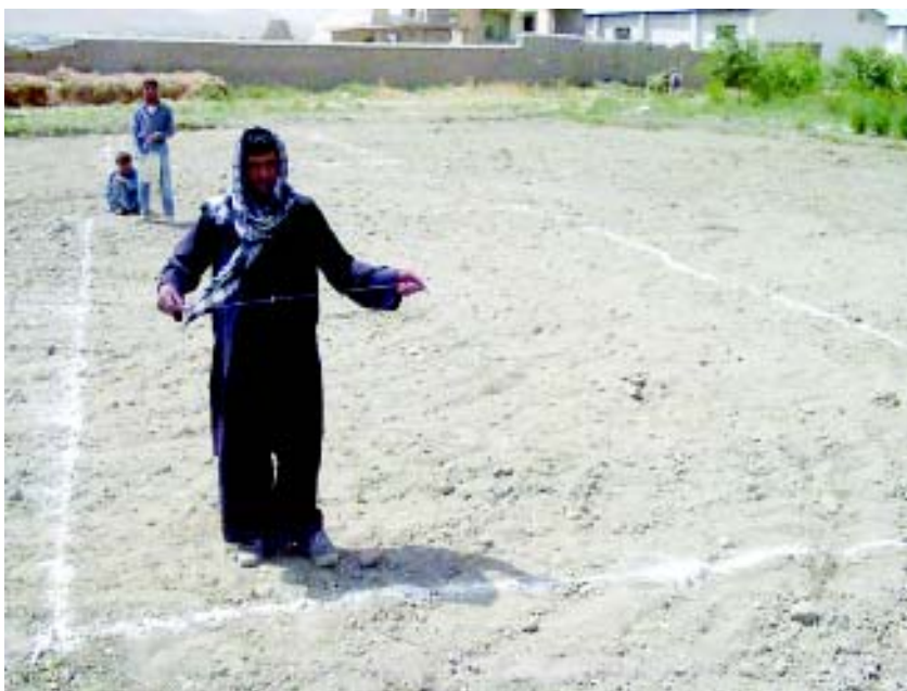
Figure 31: Marking the position of the walls
