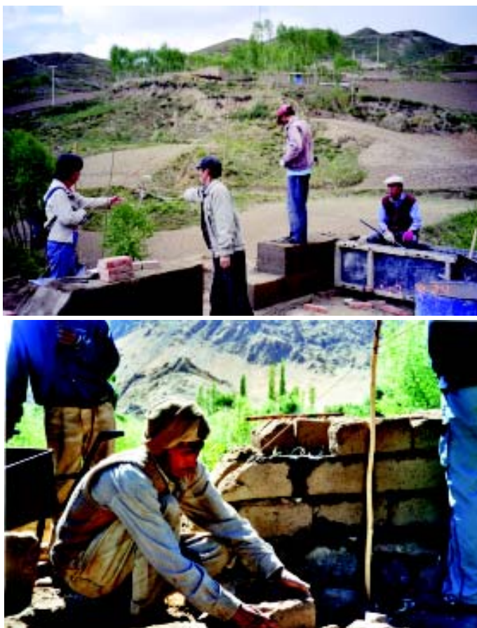
Figures 33, 34: Outlining the position of the top of the wall with thick string (in Qinghai and Ladakh)
