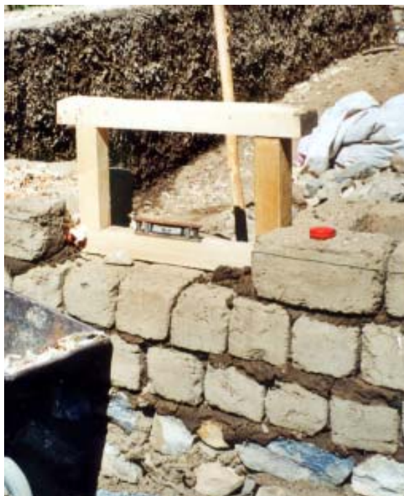
Figure 52: Positioning the shutter frame on the wall
