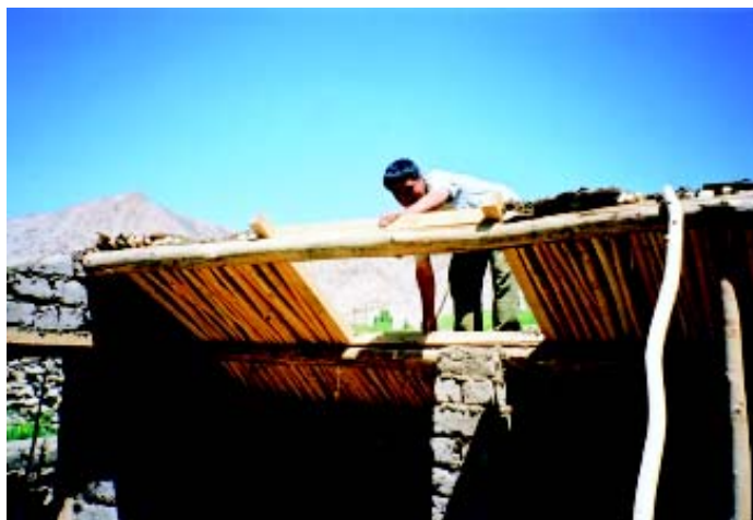
Figure 70: Fixing the frame of the roof shutter
