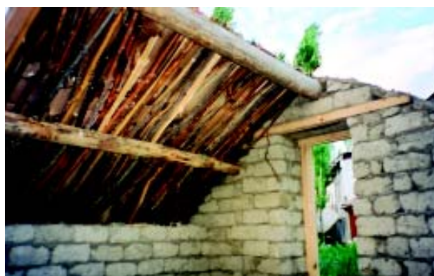
Figure 61: The layer of sticks forming the underside of the roof
