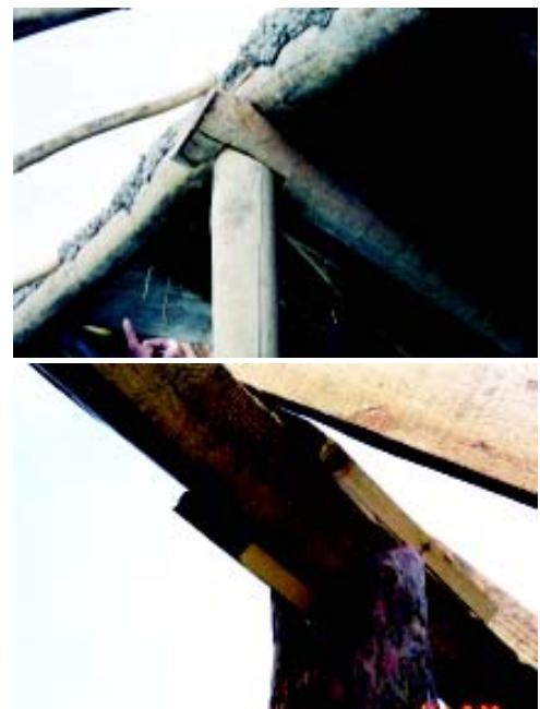
Figures 56: Fixing the beam to a post, Ladakh (top) and Qinghai (bottom)
