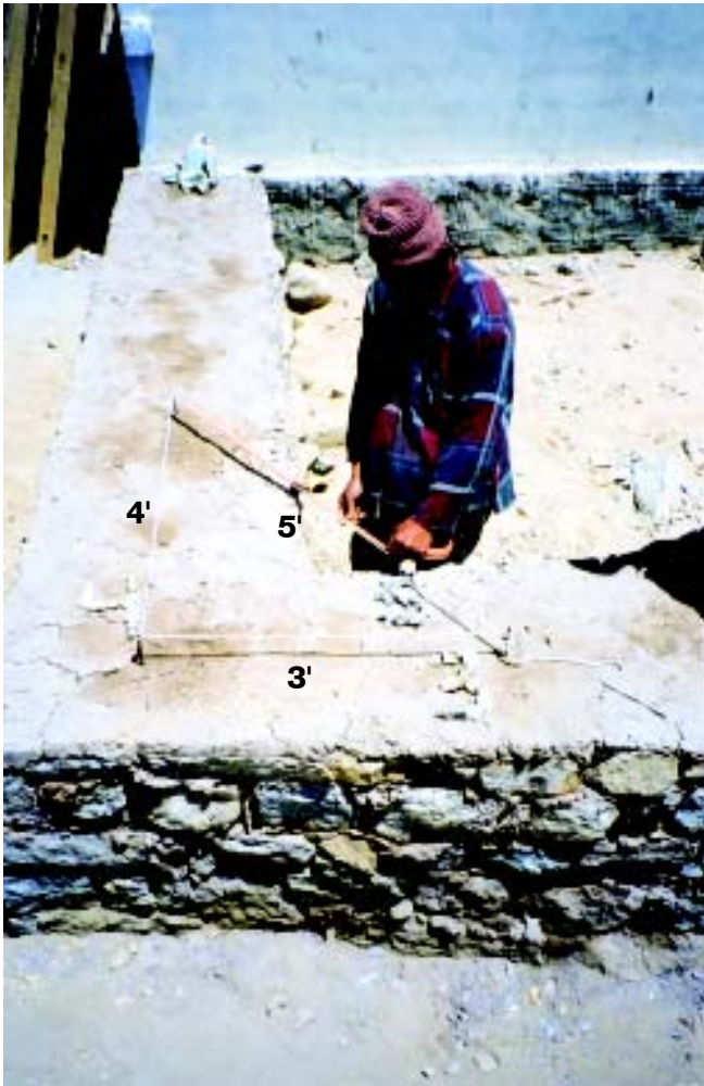
Figure 28: Drawing a right angle using the '3,4,5' method
