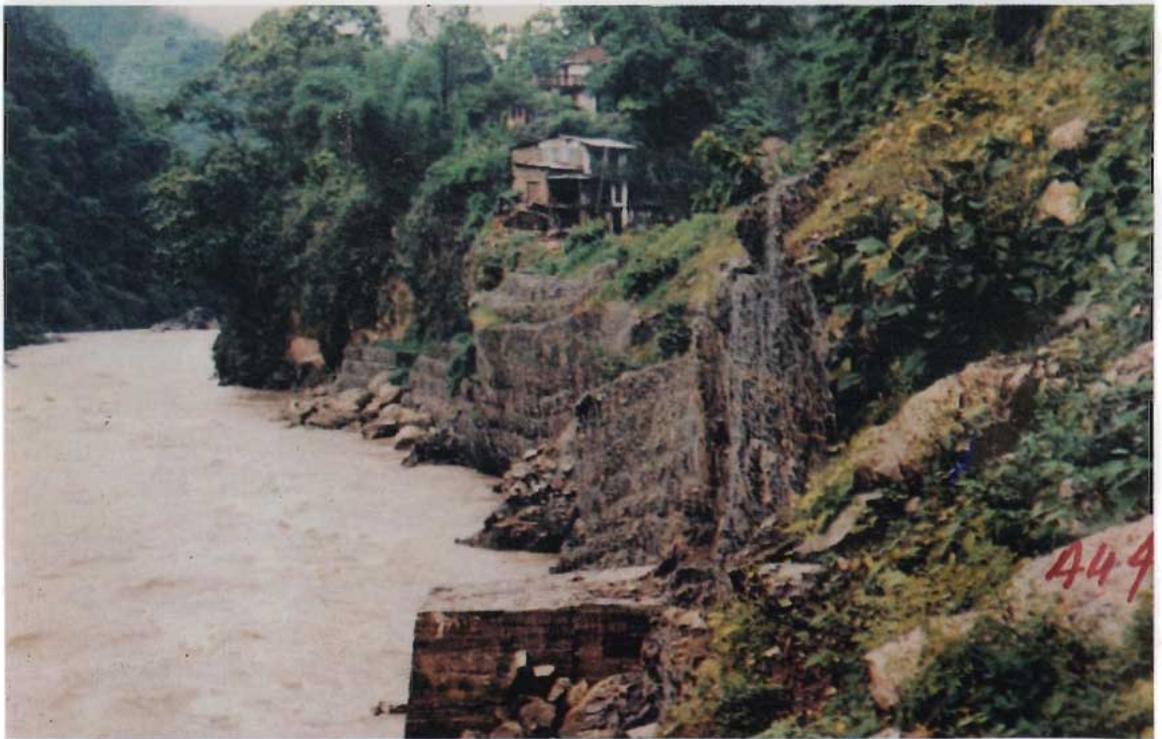
20. Improper river training work, road supporting structure without adequate foundation, Arniko Rajmarg
