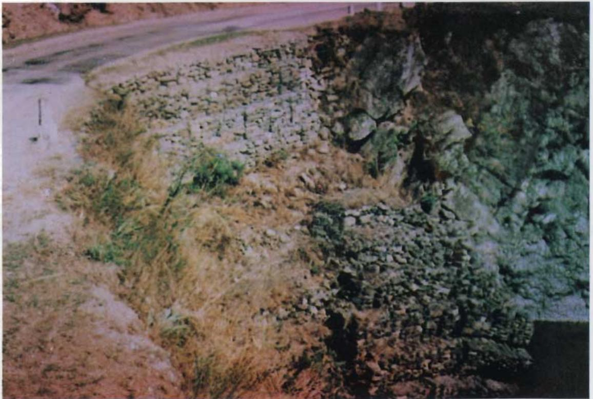
22. Improper river training work, road supporting structure without adequate foundation, Arniko Rajmarg
