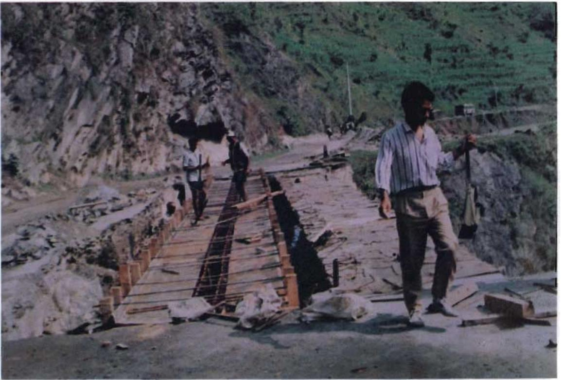
23. Construction of bridge in favourable conditions, to avoid massive river training work, improvements to Plate 22
