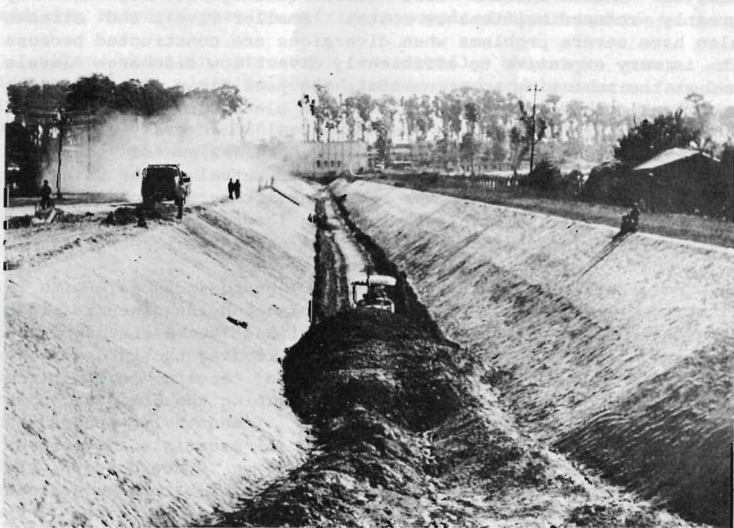
Photo XV Narayanghat, Chitwan District - Sediment removal from the main canal, Chitwan Irrigation Project. Over 2.5 meters of fine sand were deposited in this canal during the 1984 monsoon, completely blocking irrigation water flow. Better use of available data could have warned designers of such a hazard.
